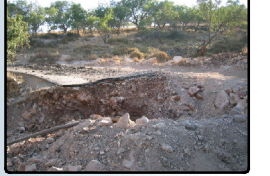
TRENCH/DITCH - A depth barrier used primarily to prevent vehicle crossing. (Nablus)
