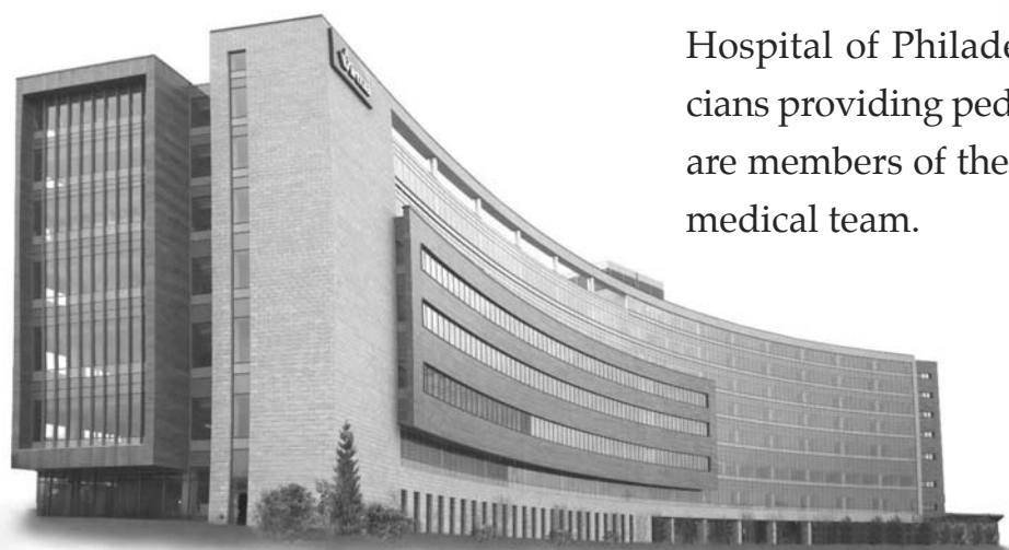
The Women and Children's pavilion at the new Virtua Voorhees hospital opening May 22, 2011.
