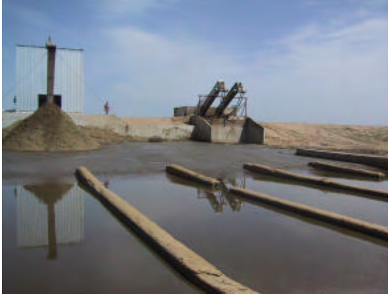
Primary Screens Background with Gravity Separators Foreground
