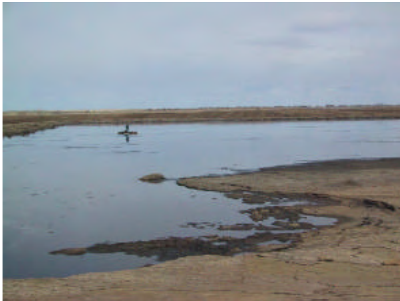
Partially Empty Primary Holding Pond Showing Sediment
