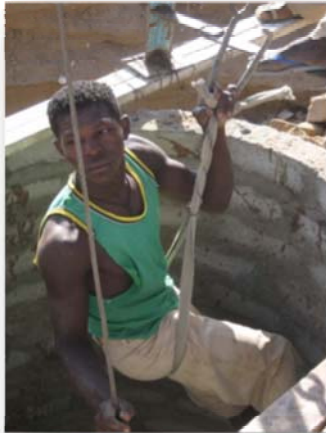
Fig.5: Lining the well in Oudi
