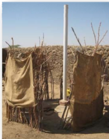
Fig.14: VIP household latrine in Darasta
