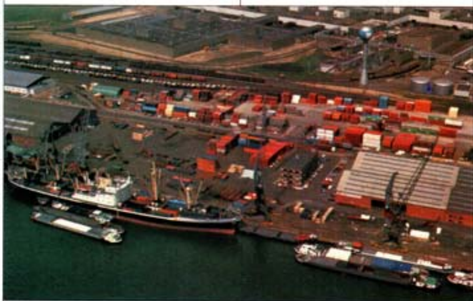
General cargo facilities are predominant in the port. In the background is one of the two large General Motors car assembly plants in the port area.
