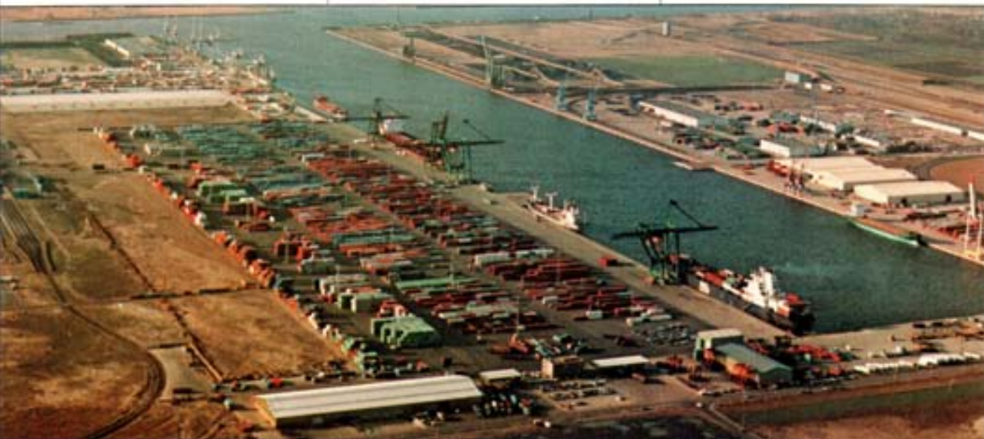
Antwerp's latest dock, inaugurated in 1982 as Delwaide Dock, has 4.7 km of quaylength and recorded a cargo turnover of 15 million tons in 1984. It hosts four container terminals and one bulk terminal. (Photograph G. Coolens)
