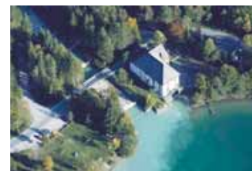
Niedernach power plant (4)
