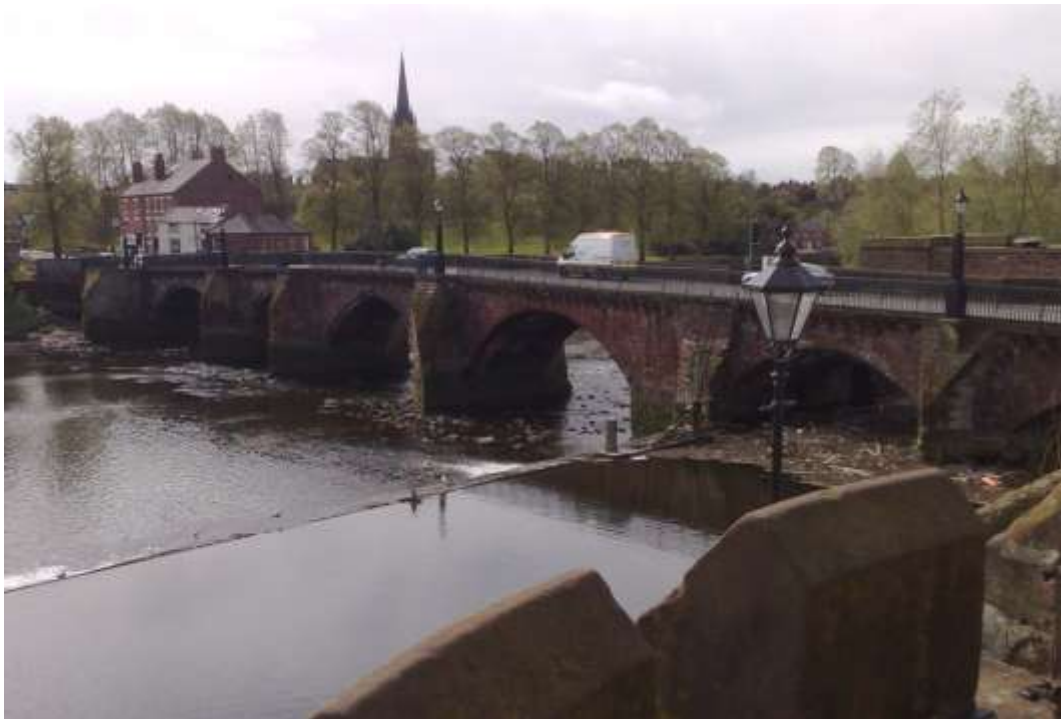
The bridge over the River Dee at Chester
