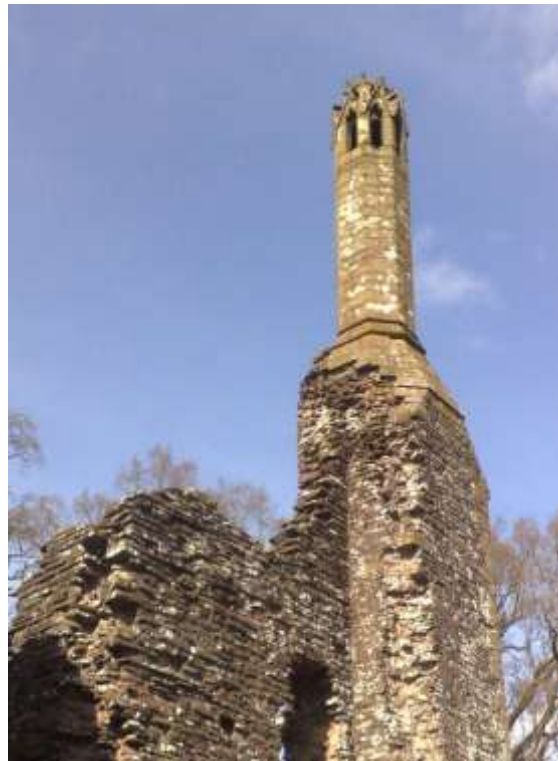
The fourteenth century chimney at Grosmont castle
