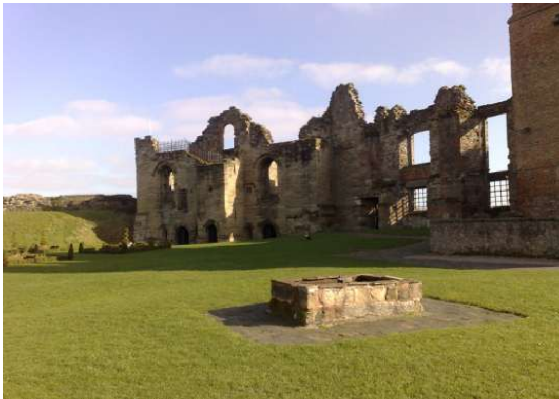
The South Tower at Tutbury
