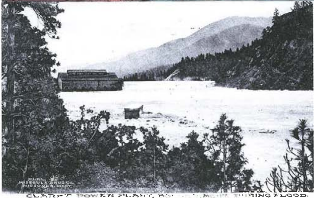
Clark's Dam (Milltown Dam)
