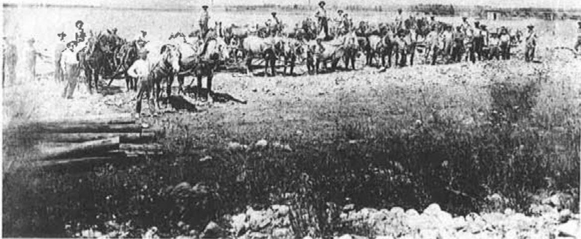
Laying the tracks for Missoula's streetcar line to Fort Missoula
