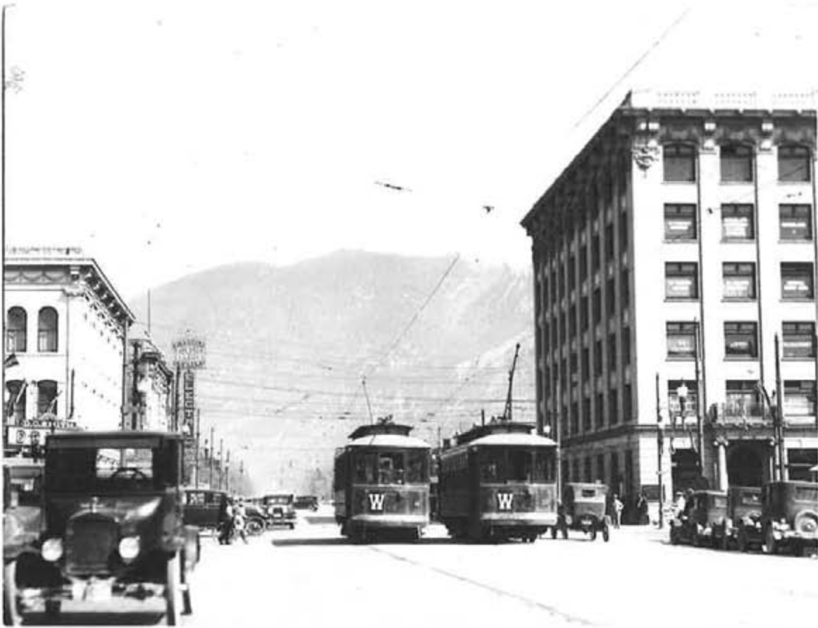
Double track along Cedar (Broadway) allowed the trolley line to serve the "West Side" of Missoula
