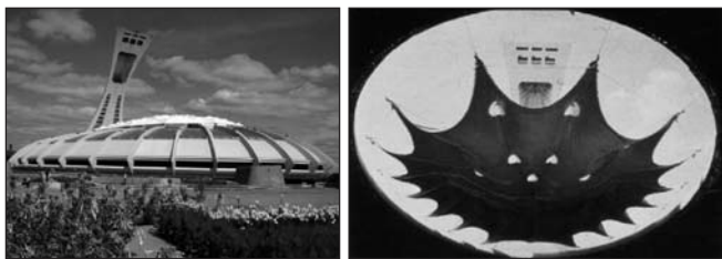
Fig. 23: Olympic Stadium in Montreal (architect: Roger Taillibert) (Olympic) an its original retractable membrane roof (Barnes, 2000)
