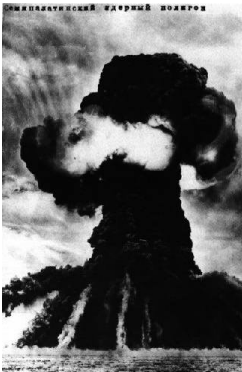
Figure 9. The Soviet nuclear explosion, “Shagan,” of 15 January 1965, designed to create a crater and dam a water reservoir.
