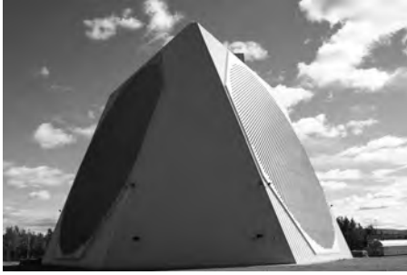
Figure 19-6. Tracking radar at Clear AFS. (USAF photo)
