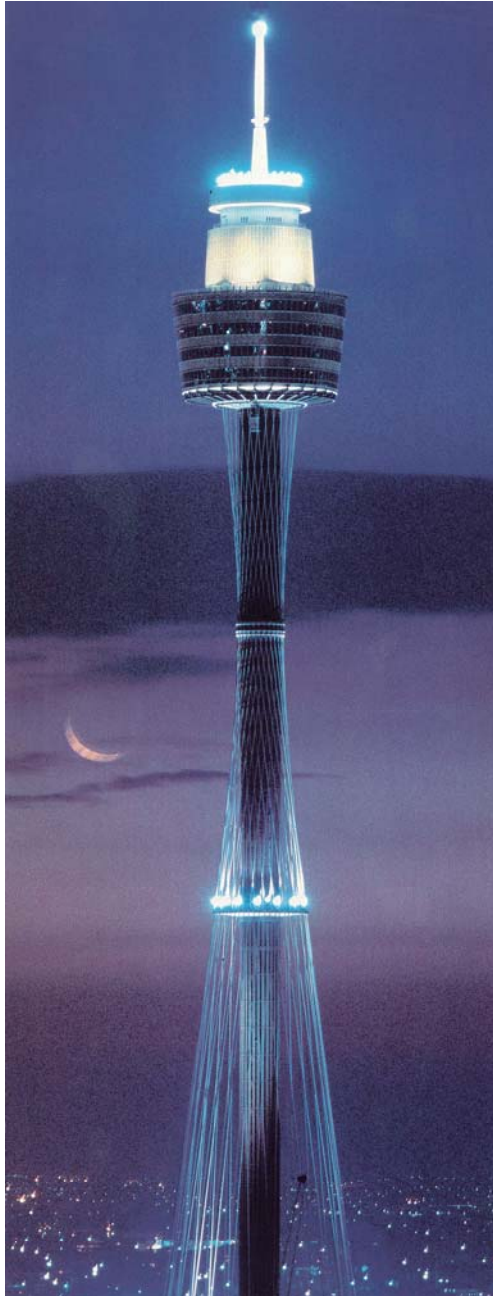
Centre Point Tower Australia (1978)
