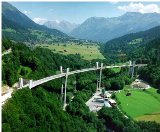
Sunniberg Bridge Switzerland (2005)
