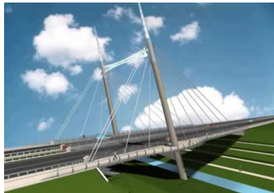
Ormiston Road Bridge New Zealand (anticipated 2007)
