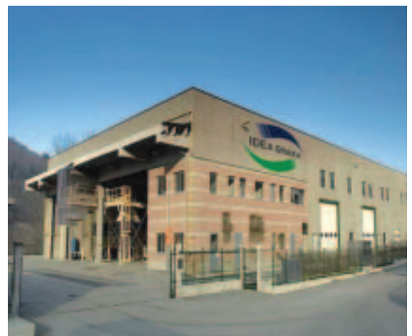
VIEW OF IDEA GRANDA PLANT IN ROCCAIONE, CUNEO
