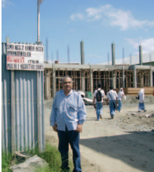
RECONSTRUCTION WORK IN BANDA ACEH THANKS TO MY TIME FOR INDONESIA
