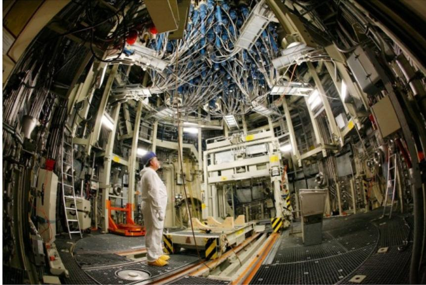
Figure 60. Control rod drives at the bottom of the Krümmel BWR reactor near Hamburg, Germany that went into operation in 1984.
