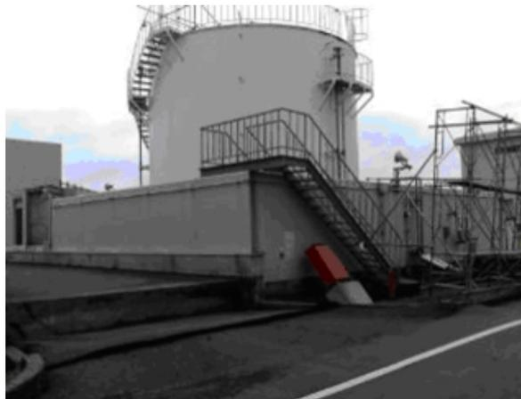
Figure 14. Earthquake-caused ground subsistence around light oil storage tank of 30,000-40,000 gallons capacity, 1979. Source: Tepco.
