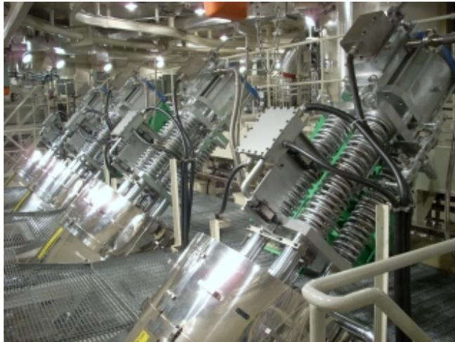
Figure 8. BWR Main Steam Isolation Valves, MSIVs. Source: Tepco.
