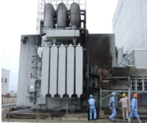
Figure 18. Transformer fire caused by 1979 earthquake. Notice the location of the transformer outside the plant enclosure and its vulnerability to water-flooding from the tsunami event.
