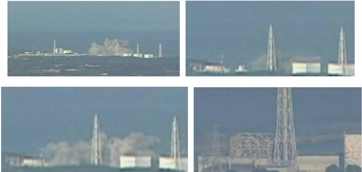
Figure 33. Fukushima Daiichi unit 1 Boiling Water Reactor, BWR nuclear power plant horizontally propagating hydrogen explosion, initiated by depressurization and steam venting, sequence of events. March 12, 2011.
