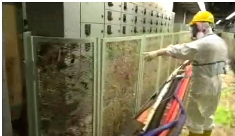
Figure 24. Tsunami water flooding of electrical switching components in basement of unit 1, May 6, 2011. Source: Tepco.
