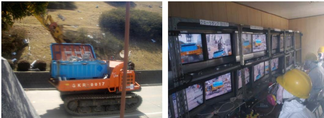
Figure 52. Removal of debris using remote control equipment and autonomous transporters. A useful design feature at the Fukushima site is an emergency command control center in an earthquake proof bunker with power supplies, radiation shielding thick walls, communication gear, food and water supplies and two air filtration systems. Source: Tepco.
