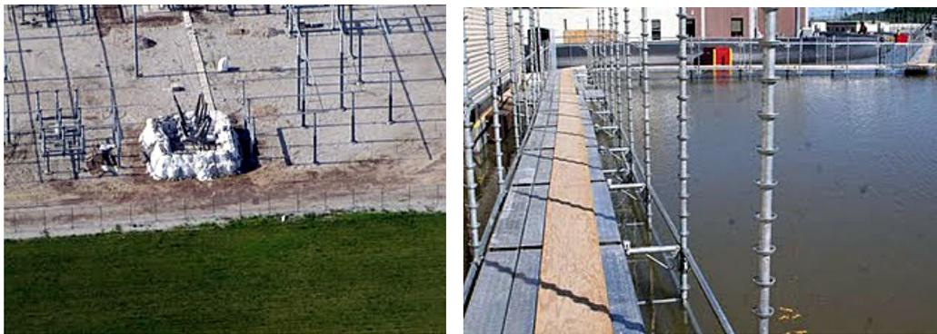
Figure 59. Circuit breaker 345 kV at transformer substation protected with sandbags and walking bridges around buildings were implemented against flooding at Fort Calhoun, Nebraska, June 13, 2011. Source: OPPD.
