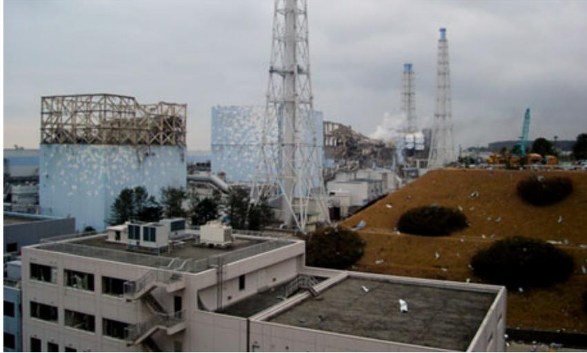
Figure 28. Damage to the upper structure of the Fukushima Daiichi unit 1, and undamaged structure of unit 2. Source: Tepco.
