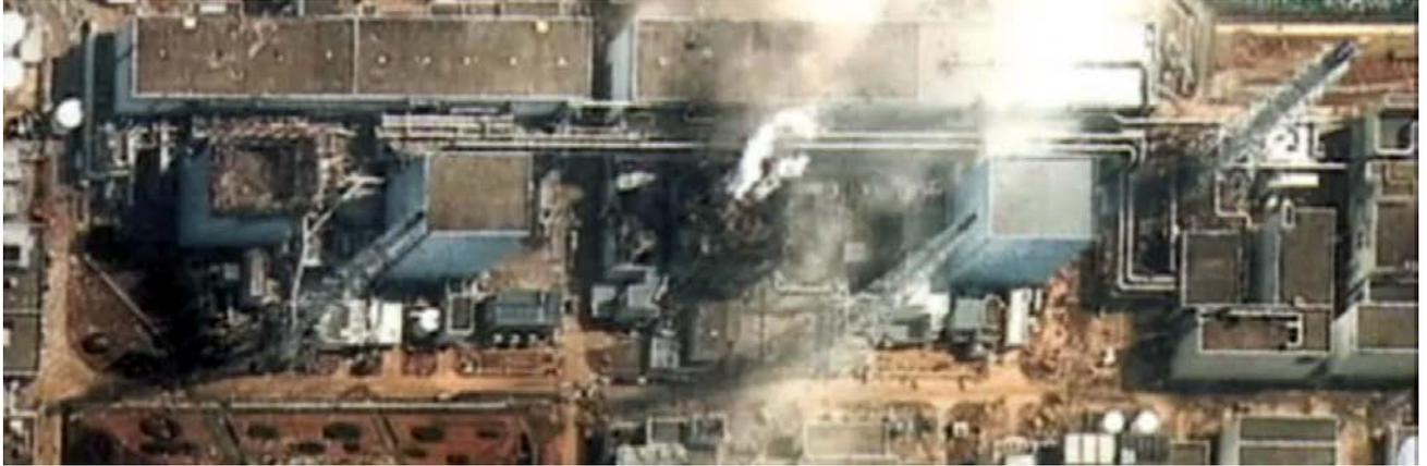
Figure 11. Remnants of a hydrogen explosion in Fukushima unit 1 (far left) exposing reactor loading deck and burying it under concrete rubble. Fire and a hydrogen explosion associated with steam depressurization and fuel damage occurred in unit 3. Fire starting at side of building in unit 4 may have originated from hydrogen generated in unit 3 that was piped into the shut-down unit 4, on March 15, 2011. Photo: DigitalGlobe.
