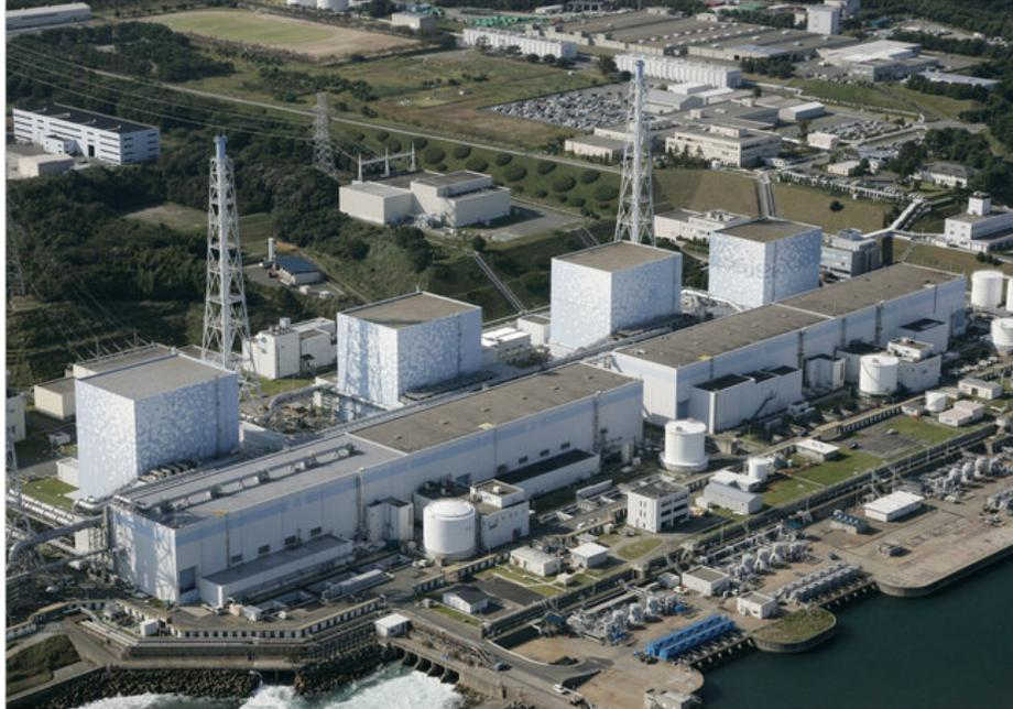
Figure 16. Fukushima Daiichi Boiling Water Reactors, BWRs nuclear Power plant, at Okumamachi, Fukushima Prefecture, Japan. The reactors are cooled with ocean water and are situated 148 miles or 238 km northeast of Tokyo. Connection to the grid shows up at the upper left side. Source: AP.
