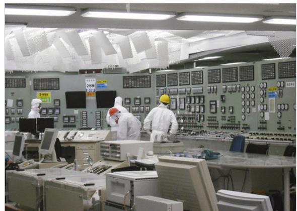
Figure 13. Station Blackout loss of power to the control room of the Fukushima Daiichi unit 1 reactor on March 24, 2011. Restoring offsite power to units 1 and 2 and power to the control room of unit 2 on March 26, 2011. The hanging ceiling tiles resulted from the earthquake. Source: Tepco.
