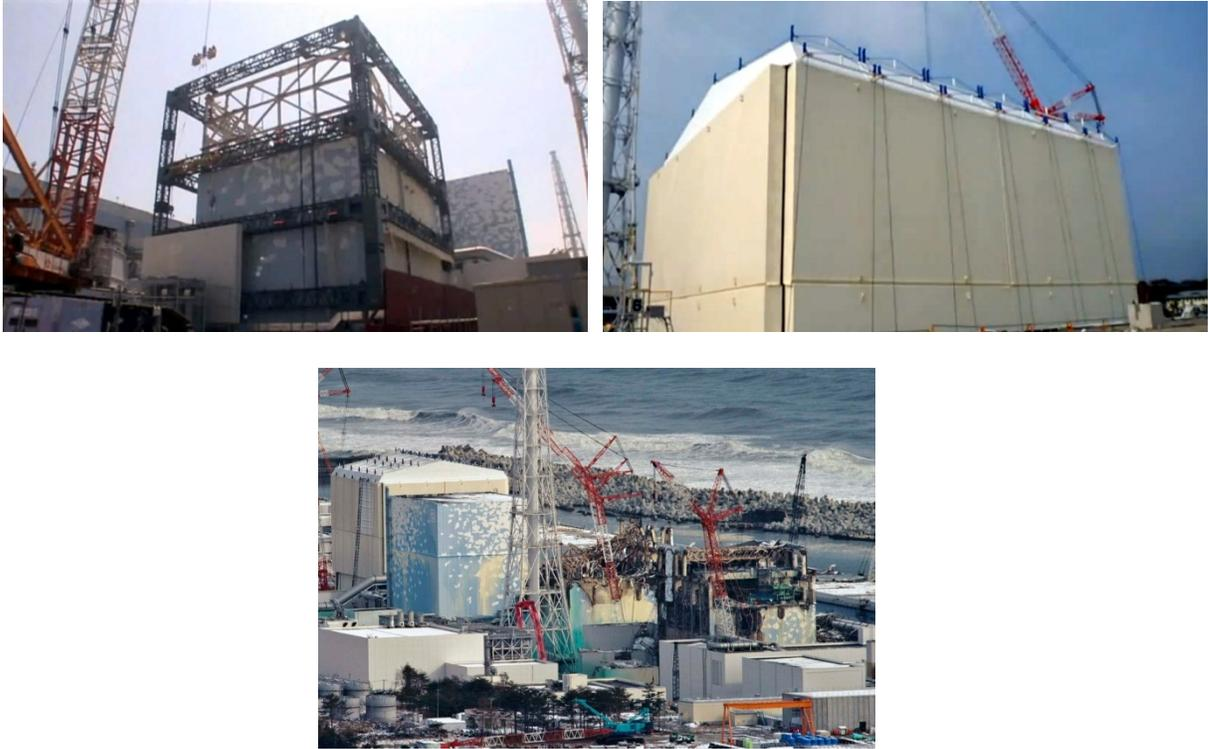
Figure 51. Encasing the Fukushima reactors.
