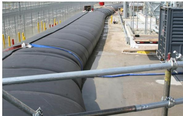
Figure 57. Fort Calhoun station, Blaine, Nebraska, 19 miles north of Omaha on the Missouri River is protected against flooding by a 2,000-ft long Aqua Dam berm from releases from the Gavins Point Dam, June 10, 2011. The berm raises the protection 6 ft above the 1,004 ft river level to the 1,010 ft Mean Sea Level, MSL. Source: OPPD.
