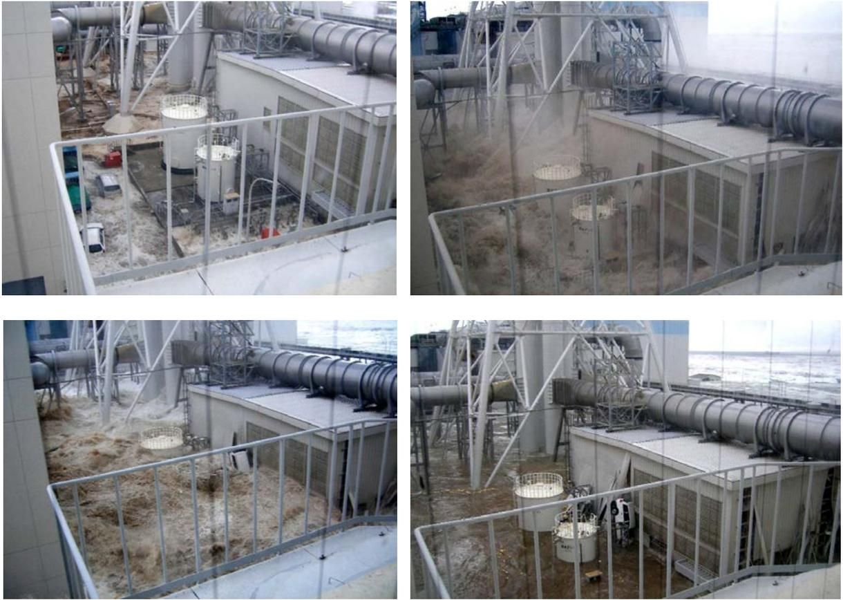
Figure 5. Fukushima Daiichi Tsunami water ingress and egress, drowning plant components at the base of the ventilation stack system, March 11, 2011. Source: Tepco.
