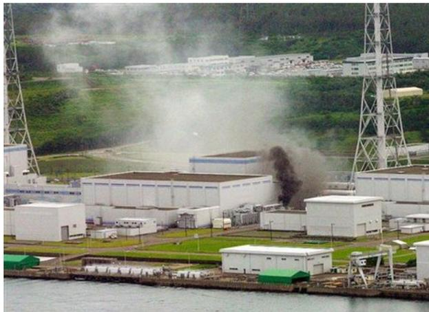
Figure 39. Burning electrical transformer resulting from the coupled earthquake and tsunami event, March 11, 2011. Source: Japan Coast Guard.
