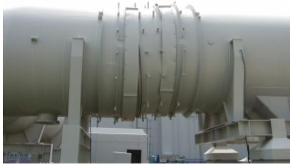
Figure 15. Earthquake-caused displacement of connecting duct to the main ventilation stack, 1979. Source: Tepco.
