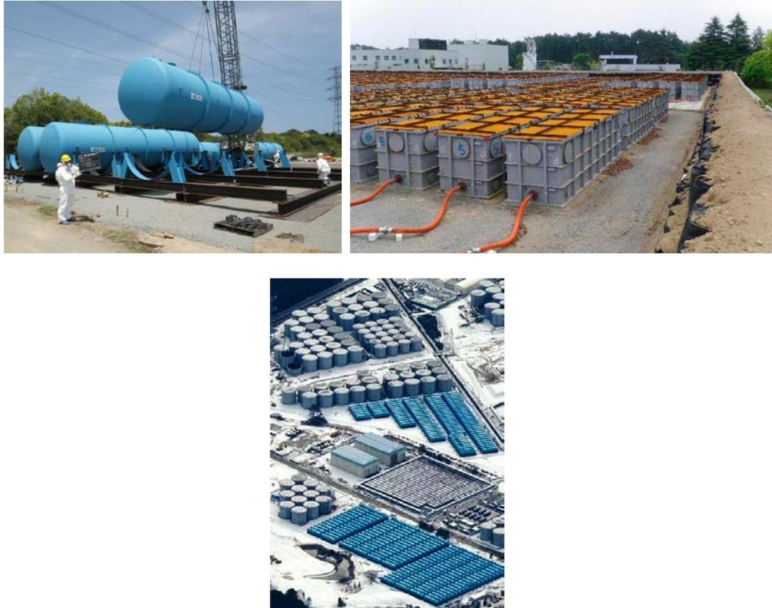
Figure 55. Storage tanks for sludge resulting from the water decontamination process and coolant storage tanks, June 10, 2011. Source: Tepco, DPA.
