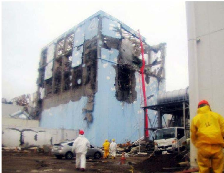
Figure 54. Damage below the fuel storage pool in unit 4 as seen from the ground on March 22, 2011. Water being pumped into the damaged spent fuel pool using a boom. Source: Tepco.
