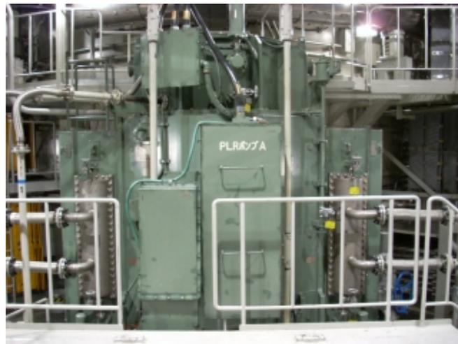
Figure 4. BWR primary coolant recirculation pump. Source: Tepco.
