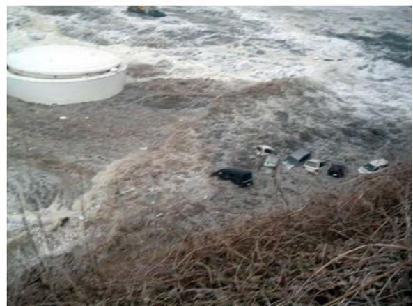
Figure 2. The tsunami wave more than 14 m (46 ft) high that originated 125 miles (200 kms) to the East, impinging on the 6 m protective wall and drowning the Fukushima Daiichi nuclear power plant site, March 11, 2011, Japan. According to the plant design, the maximum probable height of a tsunami at Fukushima was at just 5.7 meters compared with the actual 14 m. The
