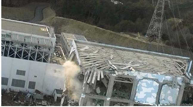
Figure 31. Fukushima Daiichi unit 4 on March 16, 17, 2011 showing steam emanating from fuel storage pool. Source: Japan Self Defense Force.
