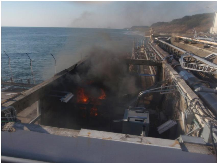
Figure 40. Fire in a battery bank initiated by a 6.3 scale aftershock on April 12, 2011. Source: Reuters.
