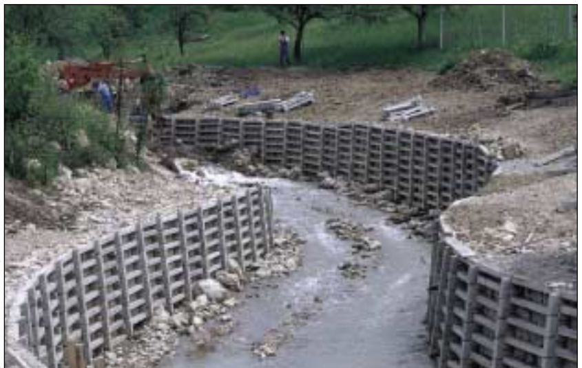
Figure 13. The Gračnica brook. Canalisation has caused drastic changes to the stream's ecosystem which has become unsuitable for most plant and animal species.
