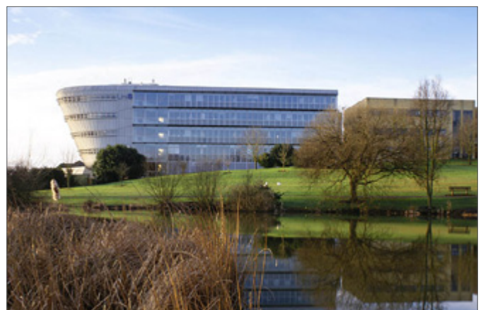
Duke of Kent building Fig. 14
