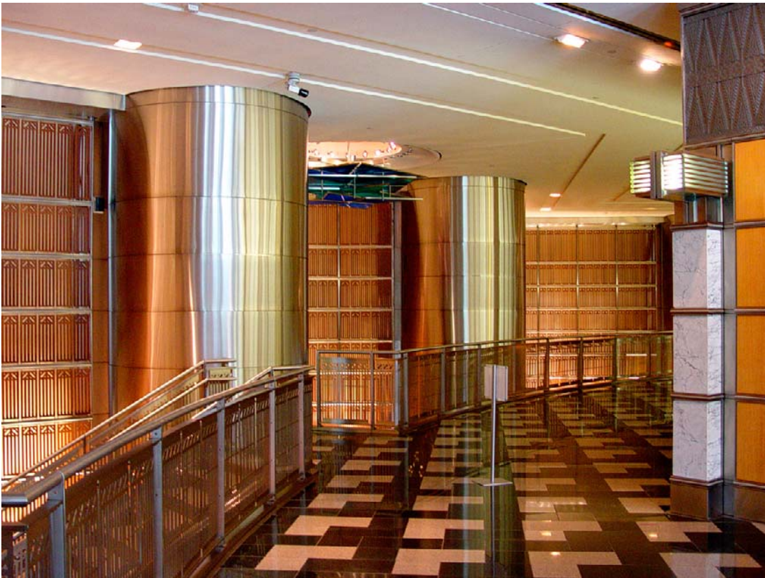
The core consists of a hollow square of walls containing elevators, mechanical shafts and other services, connected to support beams that extend out to perimeter columns.
