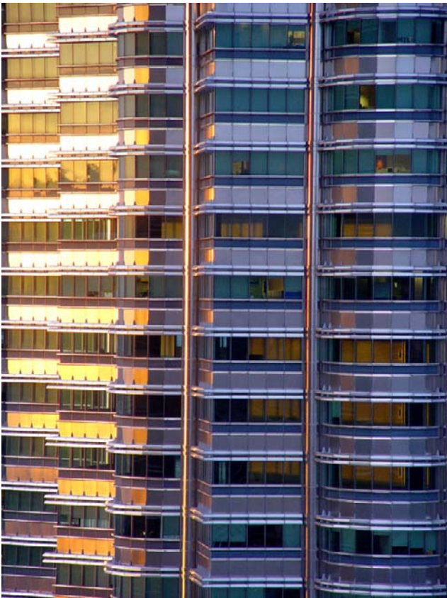
The towers and the base are clad with stainless steel extrusions and custom-made 20.38mm laminated light green glass.
