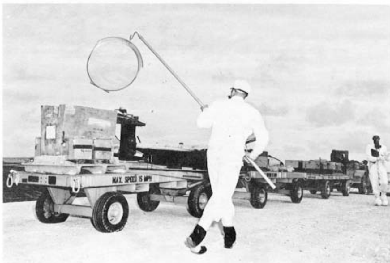
Figure 33. Filter with radioactive particulates from DOMINIC, BUMPING carried from B-57 sampler to lead cave.
