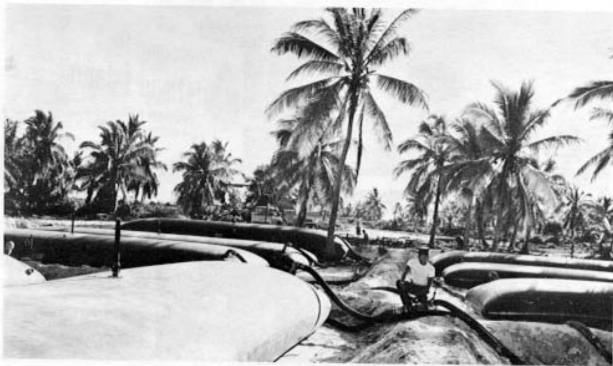
Figure 7. U.S. Marine Corps airfield fuel-dispensing system set up on Christmas Island for the DOMINIC operation.
