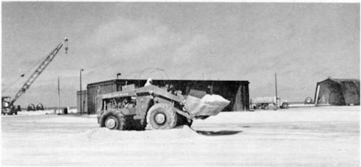
Figure 99. Loader moves contaminated soil near Thor launch pad during cleanup operations, Johnston Island, Operation DOMINIC.
