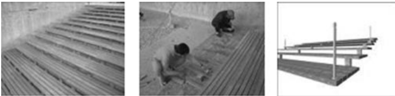
Figure 4. Preparation of the protective staircase at Persepolis.
