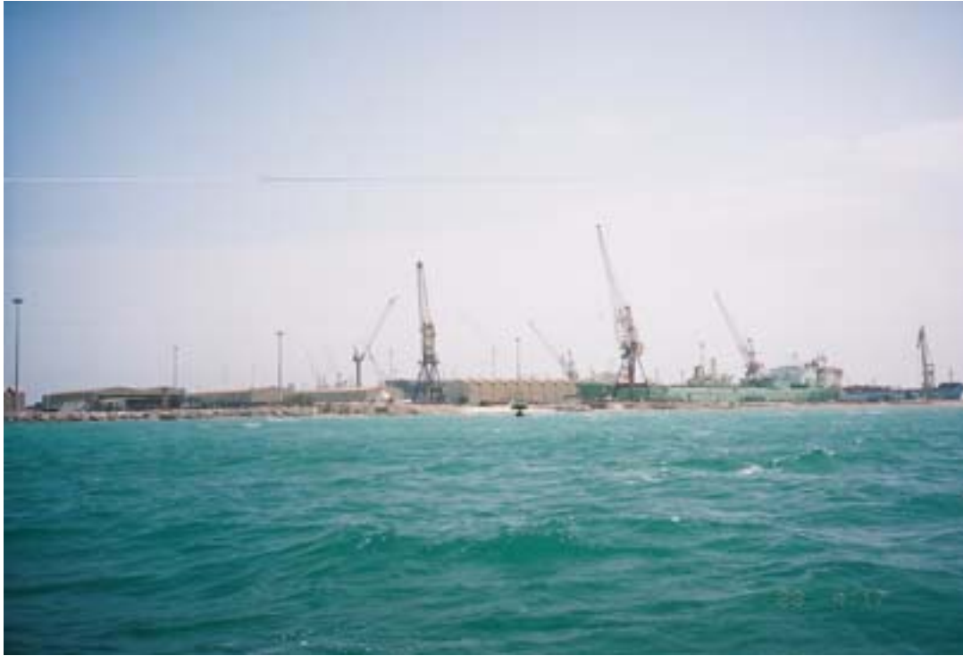
Deep Water Pier—106°54' outbound range
