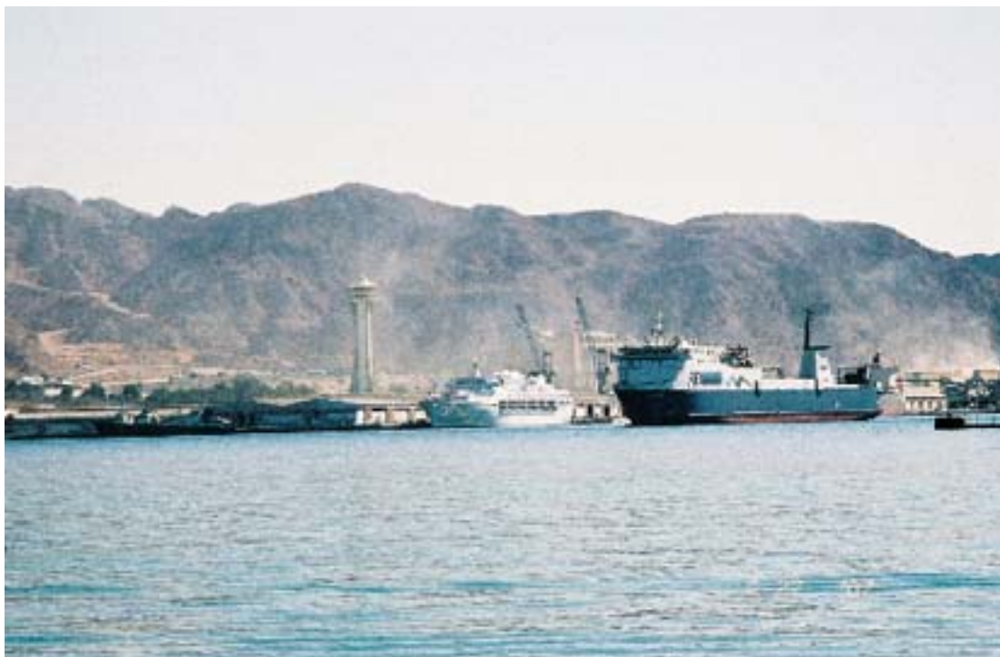
Al Aqabah—Control Tower from NW
