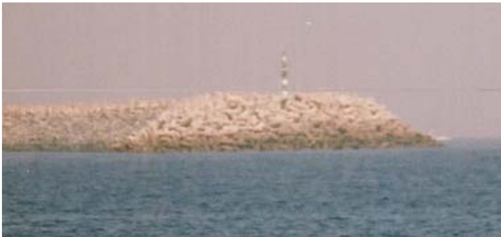
Fujayrah—South Breakwater Head
