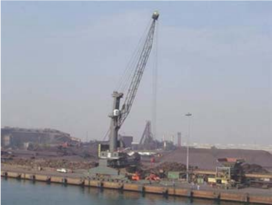
Courtesy of Qatar Petroleum Mesaieed Port Development Mesaieed—QASCO Berth No. 2
