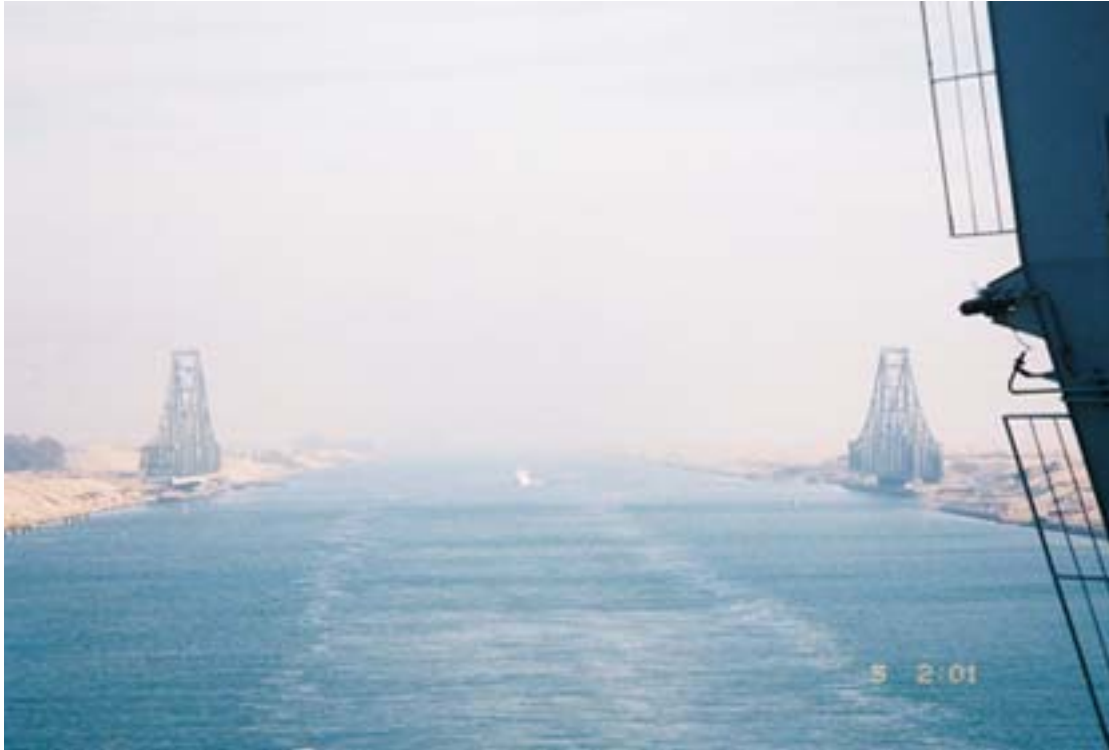
El Firdan Bridge from S
