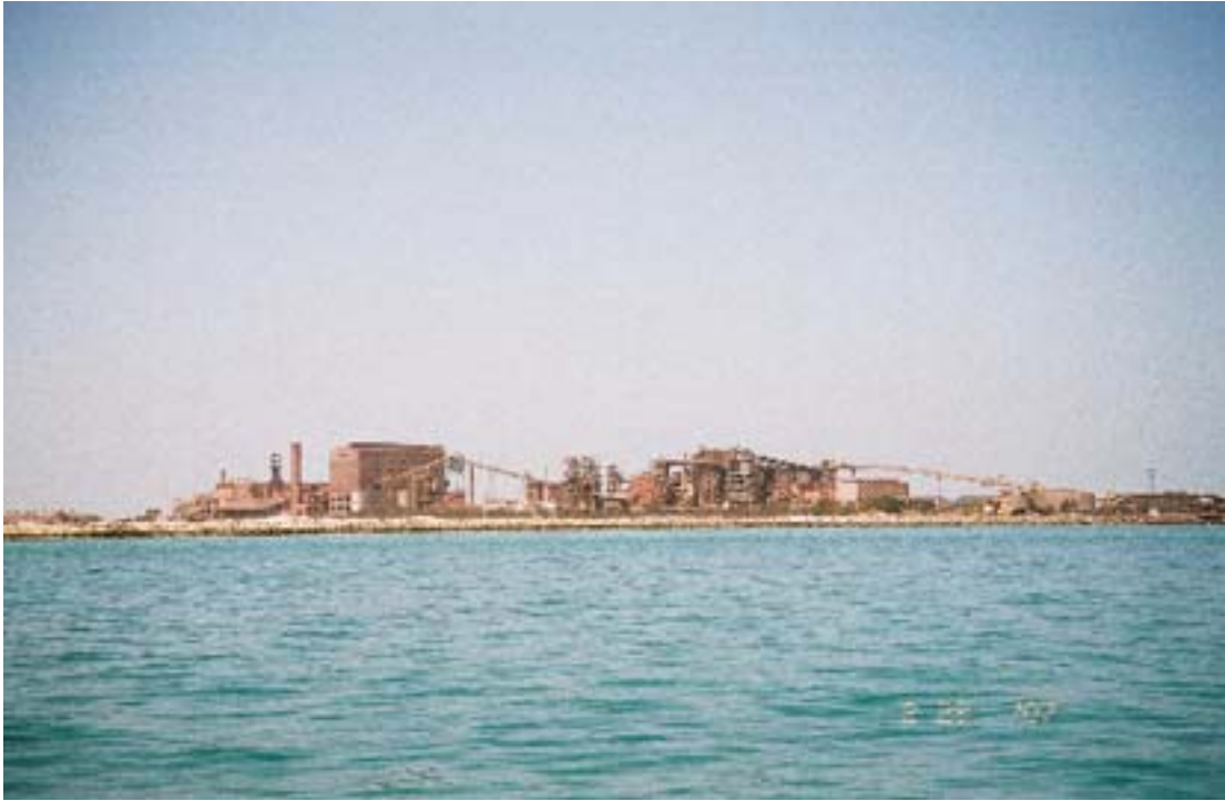
Mina Salman—GHC Plant
