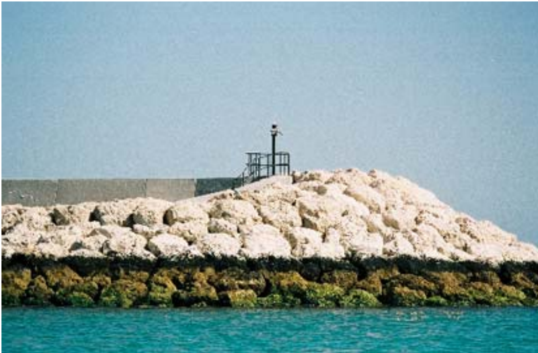
Mina Salman—Khalid Bin Salman jetty light
