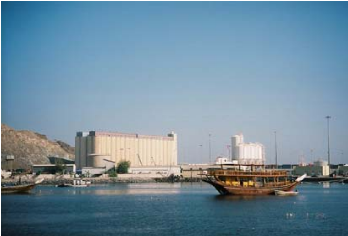
Mina Qabus—Grain Silos
