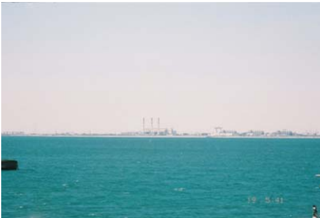
Aden Outer Harbor—Power plant chimney
