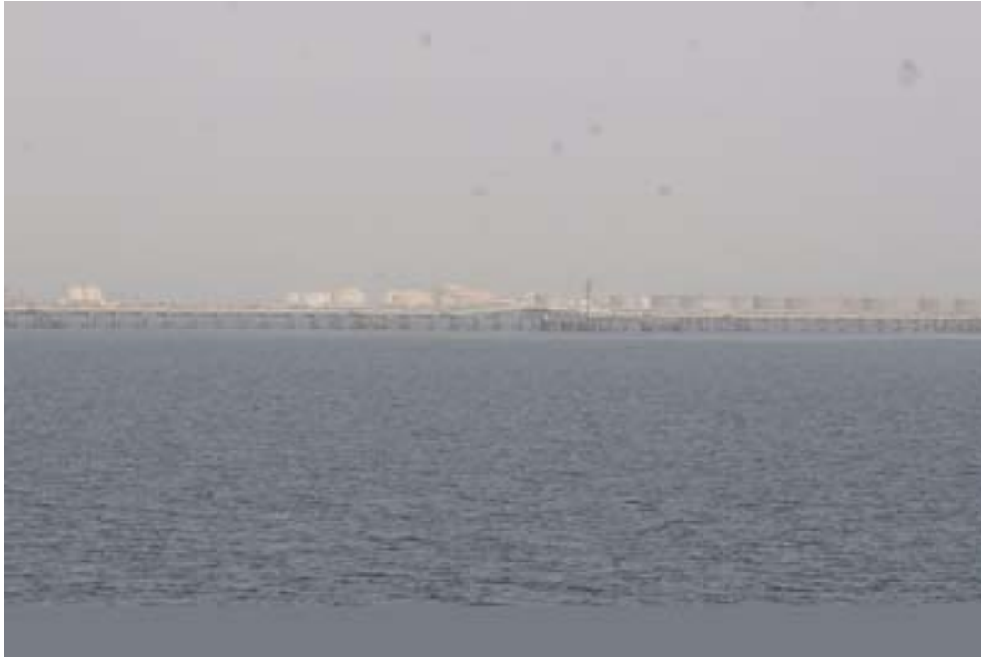
Al Jubayl—King Fahd Industrial Port Sea Tanker Terminal
