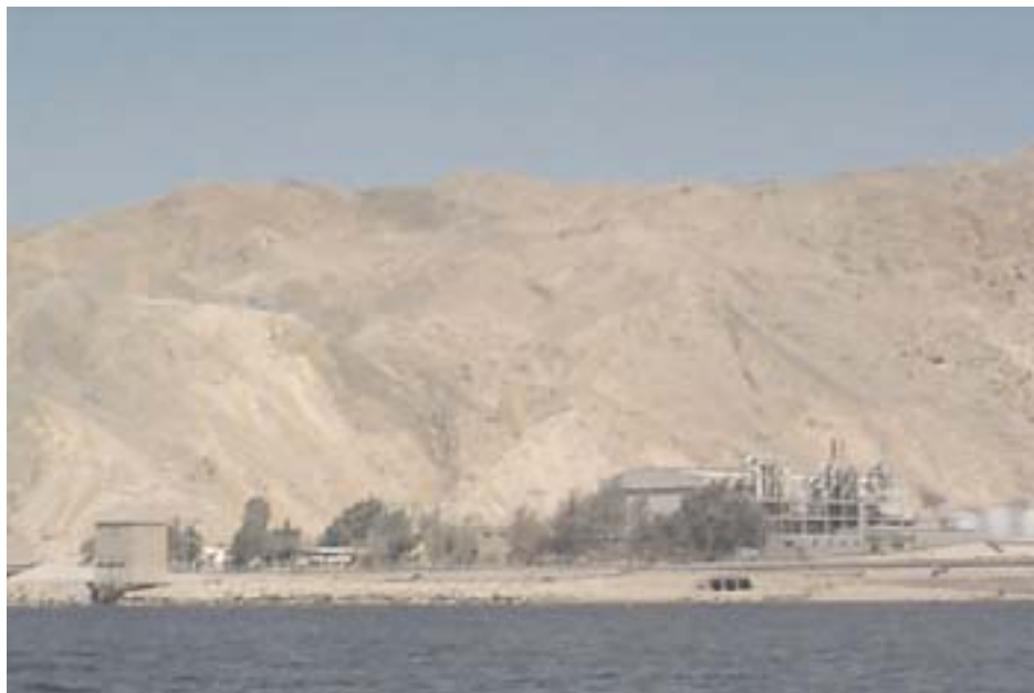
Al Aqabah—Power Station
