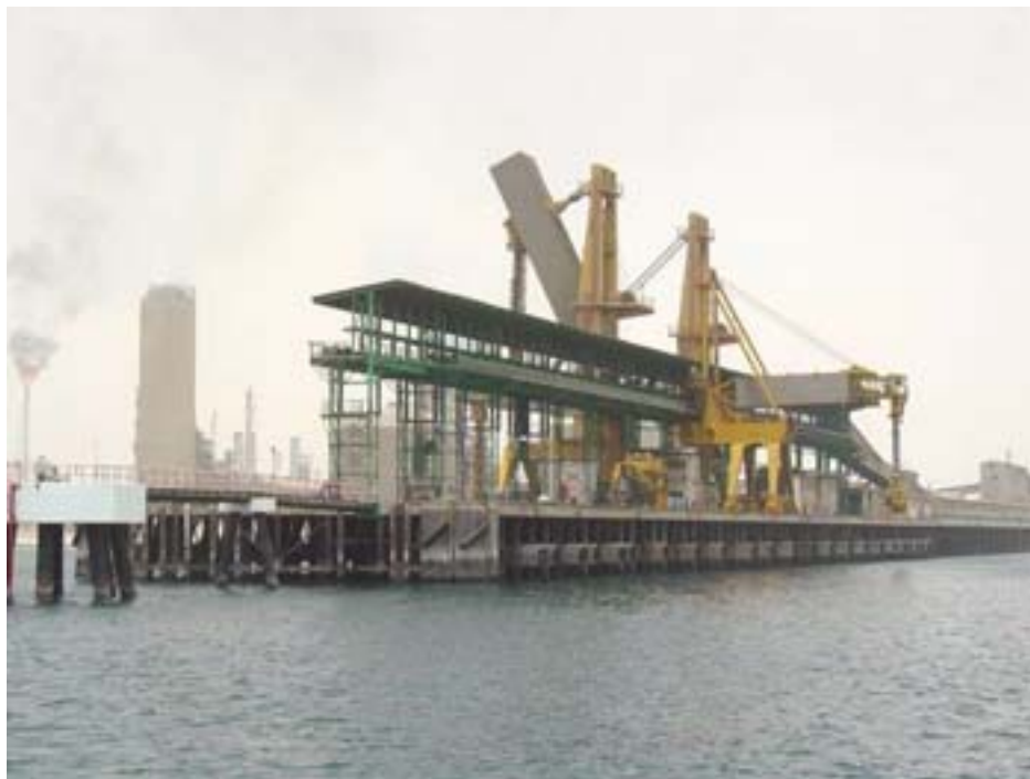
Courtesy of Qatar Petroleum Mesaieed Port Development Mesaieed—QAFCO Berth No. 1 (chartered as Berth No. 20)
