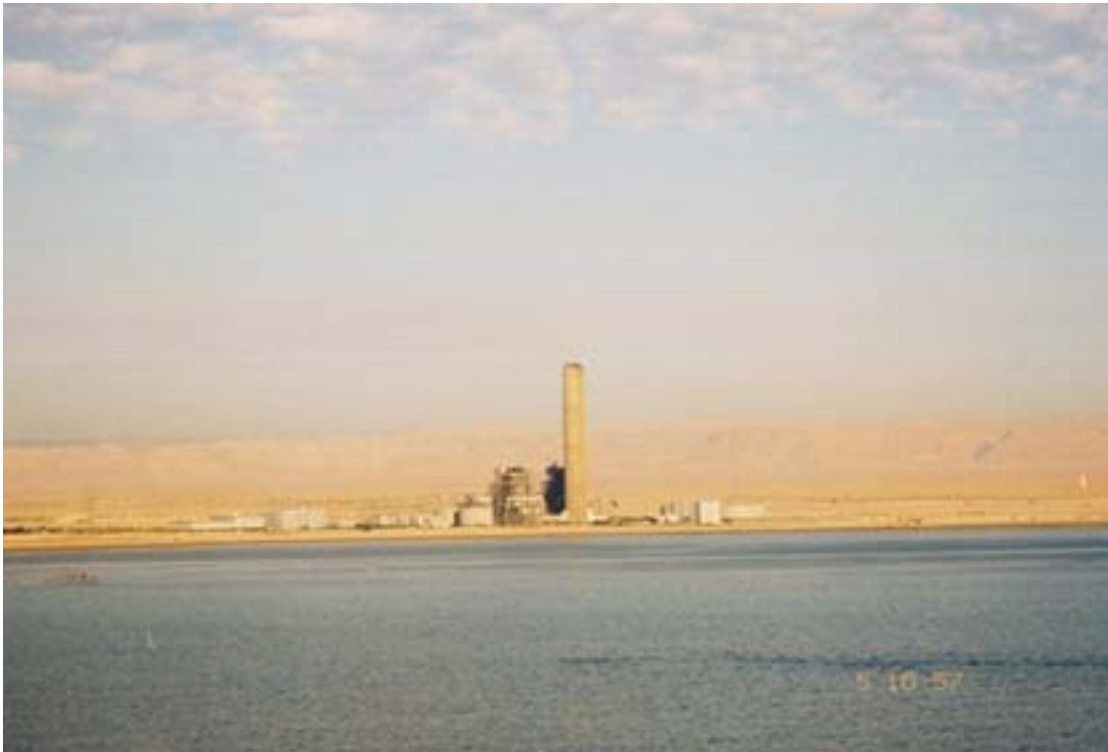
Suez Canal—Conspicuous chimney close E of South Entrance
