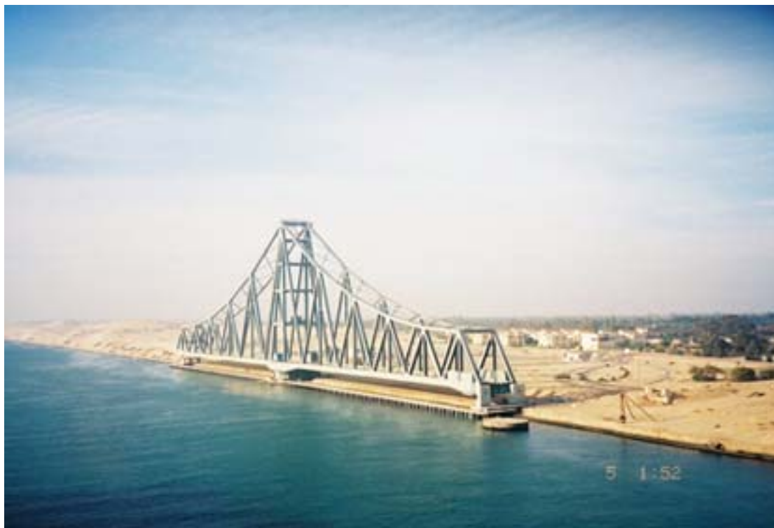
El Firdan Bridge—West bank span
