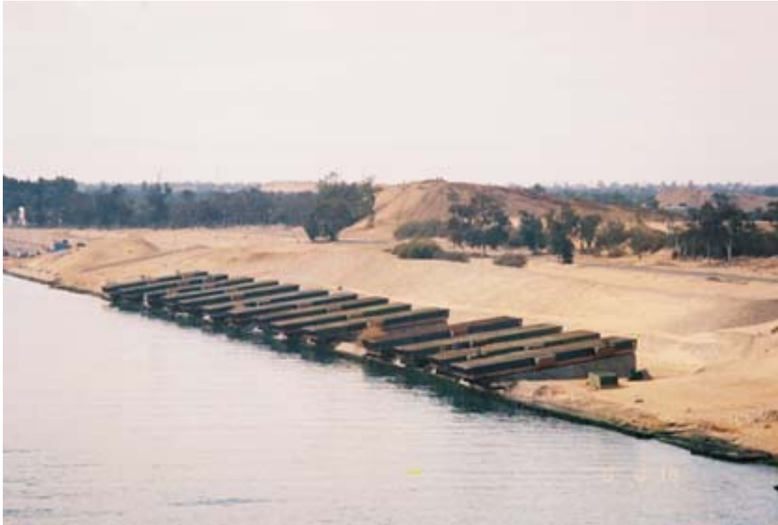
Pontoon bridge—Ready for deployment
