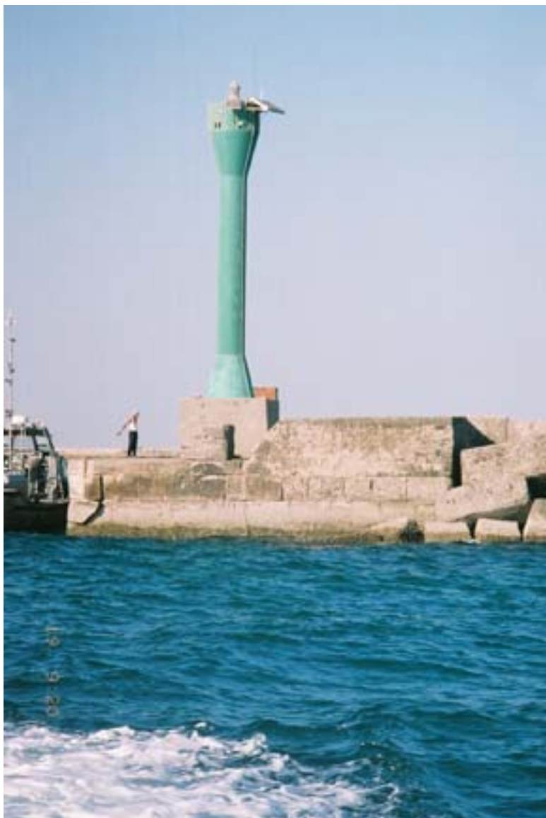
Aden—Ras Marbut (Steamer Point) Breakwater Light
