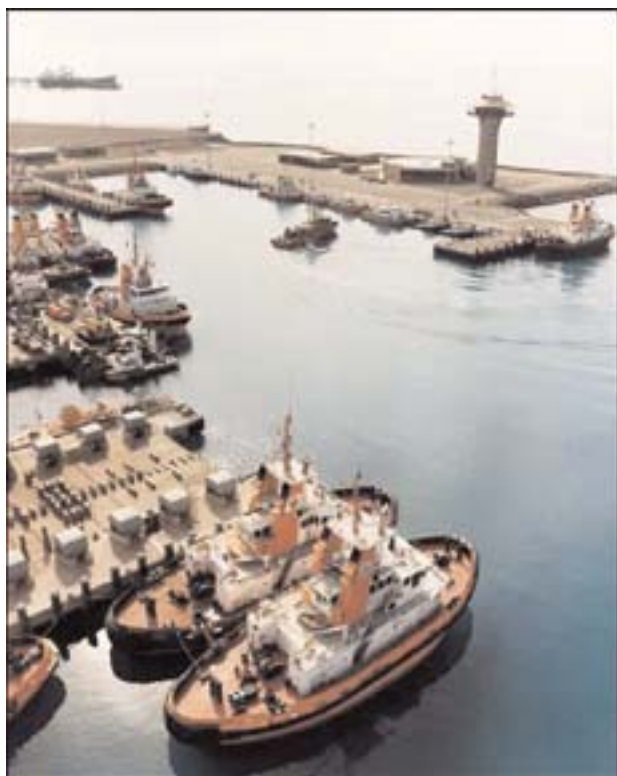
King Fahd Port Control Tower
