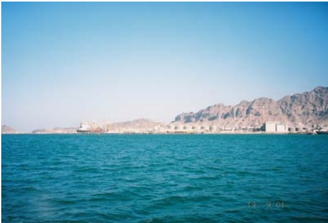
Aden Inner Harbor—Approach to Container Terminal/Home Trade Quay (left) and silos (center)
