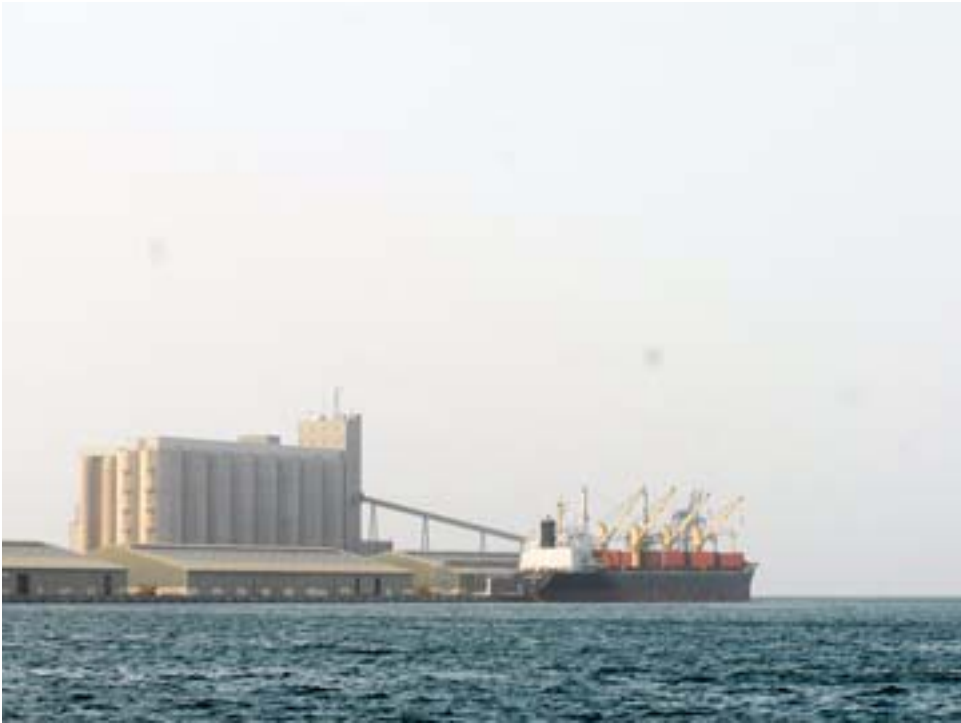
Courtesy of Abu Dhabi Ports Company Abu Dhabi—Silos at entrance to Mina Zayed
