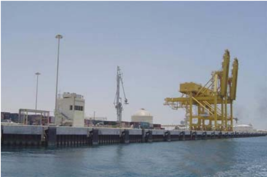
Courtesy of Qatar Petroleum Mesaieed Port Development Mesaieed—Q-CHEM Berth No. 1 and Q-CHEM Berth No. 2
