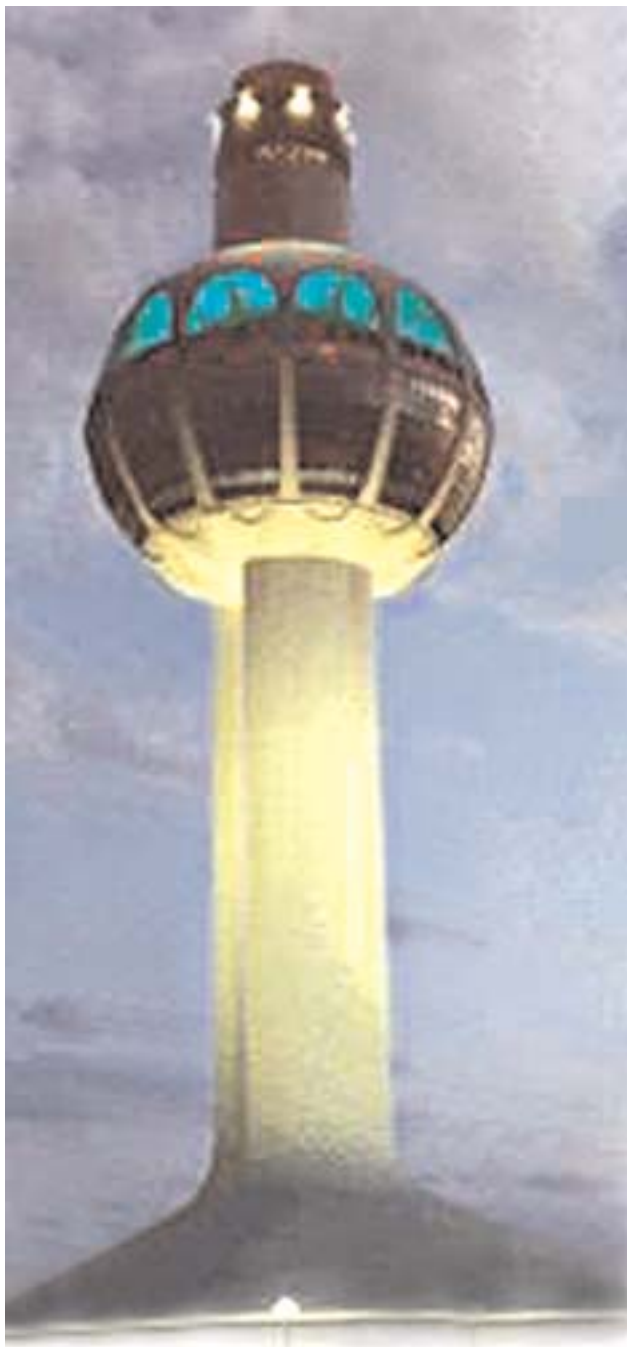
Jiddah Marine Control Tower
