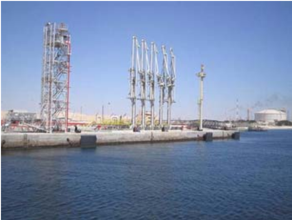
Courtesy of Qatar Petroleum Mesaieed Port Development Mesaieed—Multi-Product Berth (MPB)
