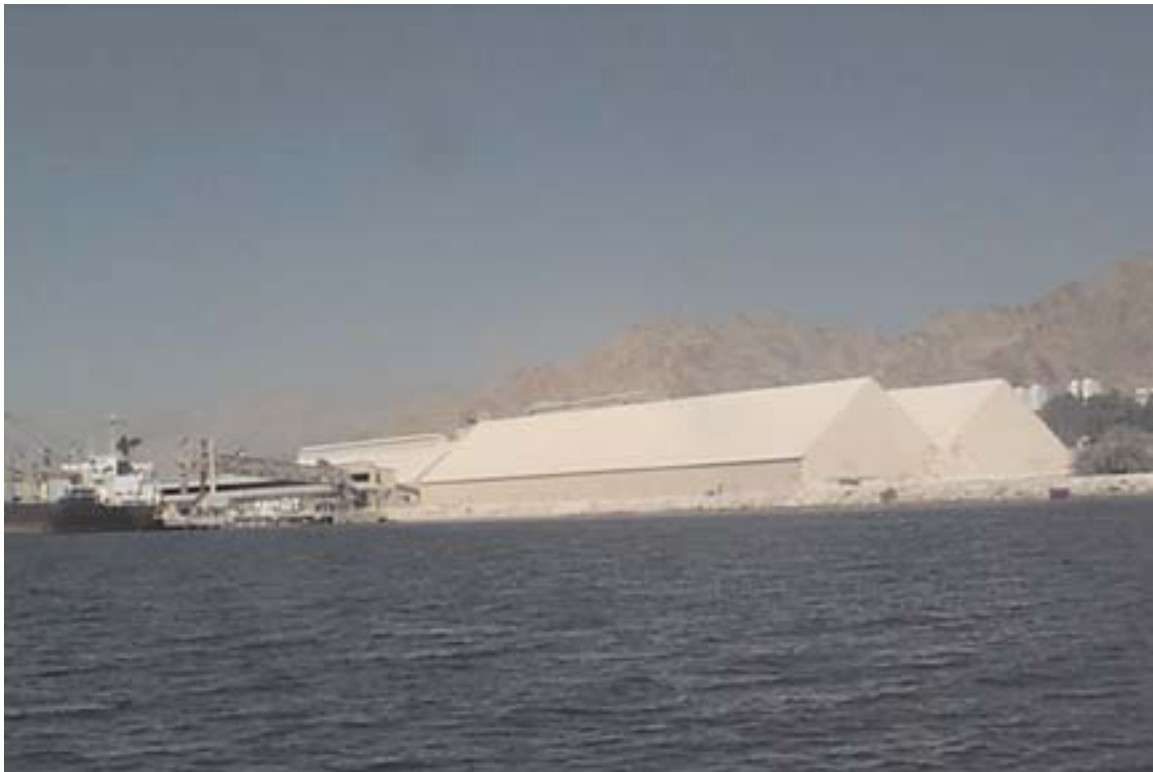
Al Aqabah—Phosphate Terminal
