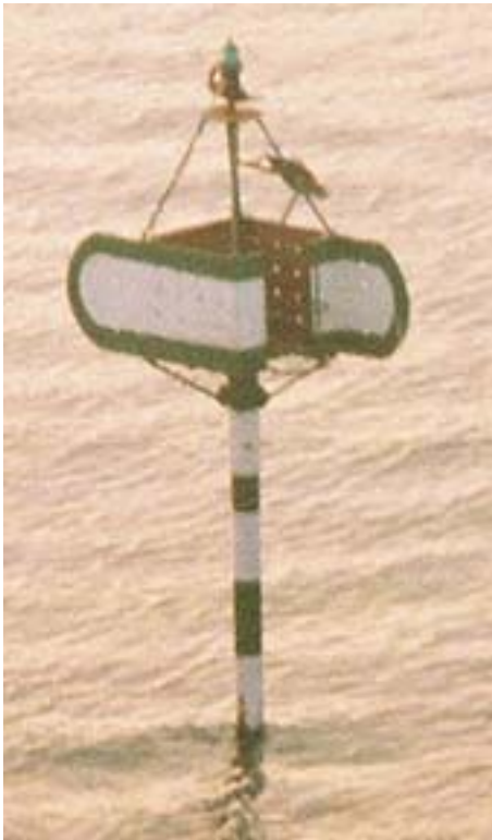
Suez Canal—Typical E side channel marker
