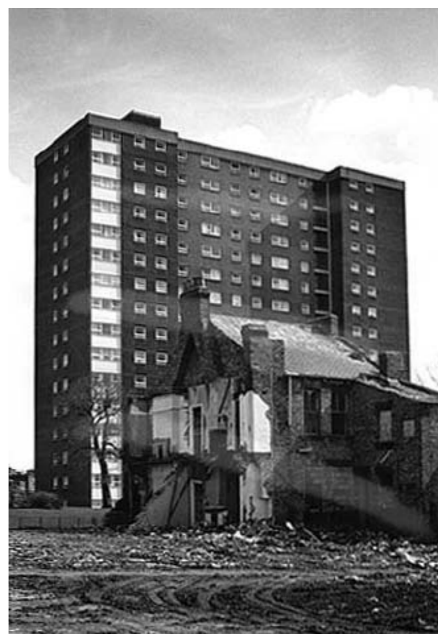
Bensham Court Flats
