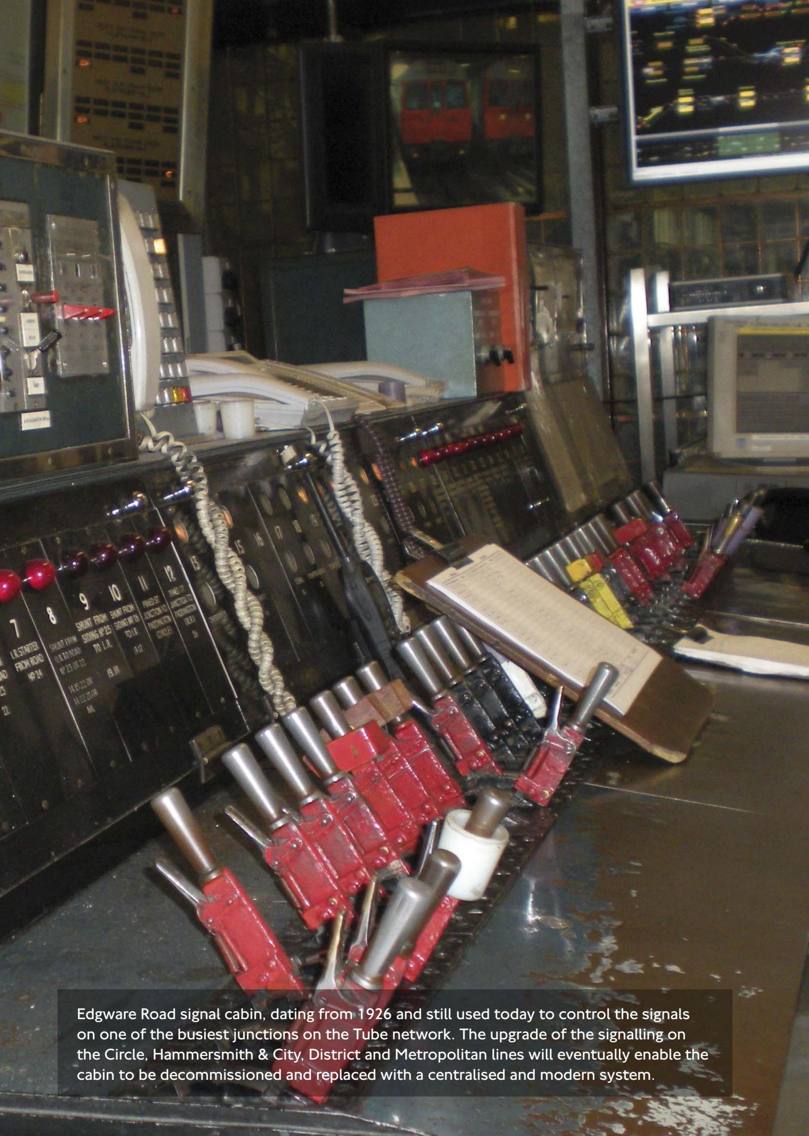
Edgware Road signal cabin, dating from 1926 and still used today to control the signals on one of the busiest junctions on the Tube network. The upgrade of the signalling on the Circle, Hammersmith & City, District and Metropolitan lines will eventually enable the cabin to be decommissioned and replaced with a centralised and modern system.
