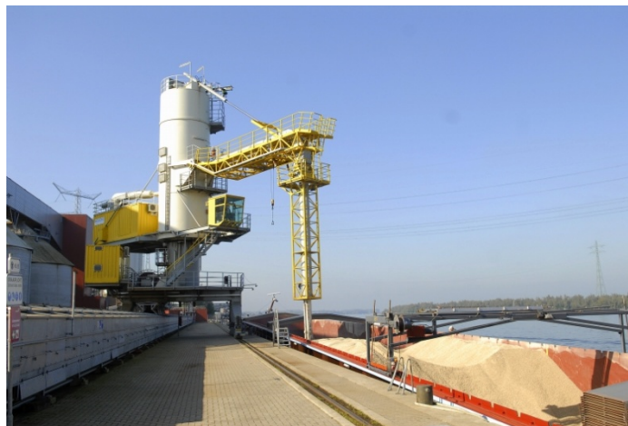
Figure 2.40 Dedicated quay at the RWE-Essent owned Amer coal power plant to unload wood pellets. It is situated at Geertruidenberg, roughly 50 km from the Rotterdam harbour. Source: Afval online (2011)
