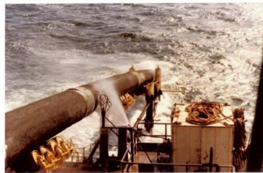
Figure 0-5 Pipelaying over the stinger
