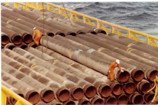
Figure 0-4 Coated pipe joints on pipe supply ship
