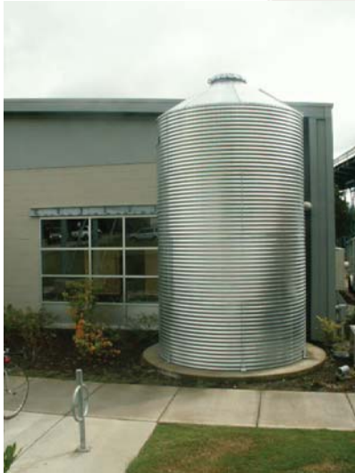
◀ This cistern illustrates a larger scale facility that may serve an office or retail establishment. The water is used to irrigate native plant landscaping at Outdoor Chattanooga.
