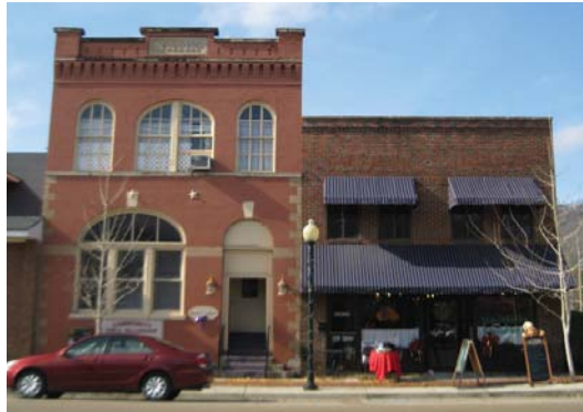
◀ Existing downtowns and neighborhood commercial districts are often good examples of mixed-use as well. These areas are prime for redevelopment as in Jasper, Tennessee where office, retail, and a cafe are all close by.
