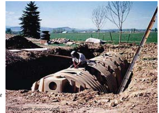
► This underground storage tank installation will be used for irrigation.
