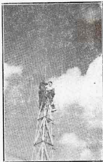
Antenna tower of KALW San Francisco Educational FM Station
