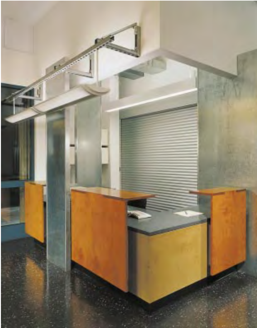
The receptionists' desk is central to the clinic's operational success. It is lighted for functionality with two fluorescent lights, one blending perforated steel and translucent diffusers; the other hanging behind the receptionist's area.
