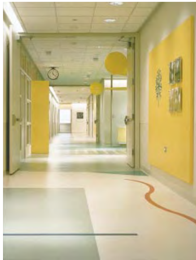
Shielded, continuous fluorescent cove fixtures were used to minimize glare.
