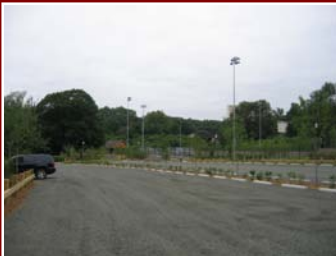
▼ ADA-compliant Access Ramps
