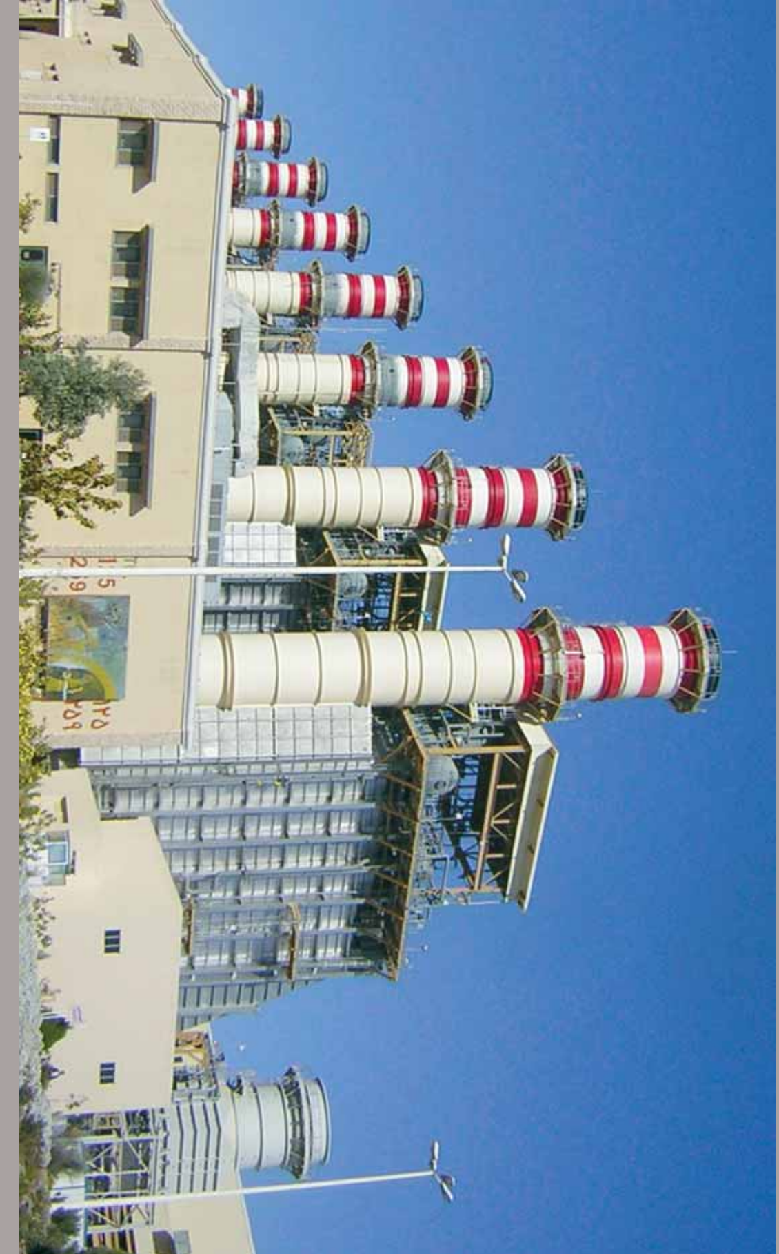
KERMAN CCPP Power Plant
