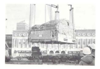
The entire vault was carefully excavated, encased in a concrete tray and lifted by giant crane in a single operation in 1986. In 1988 the vault and the bridge remains were restored to the riverside.
