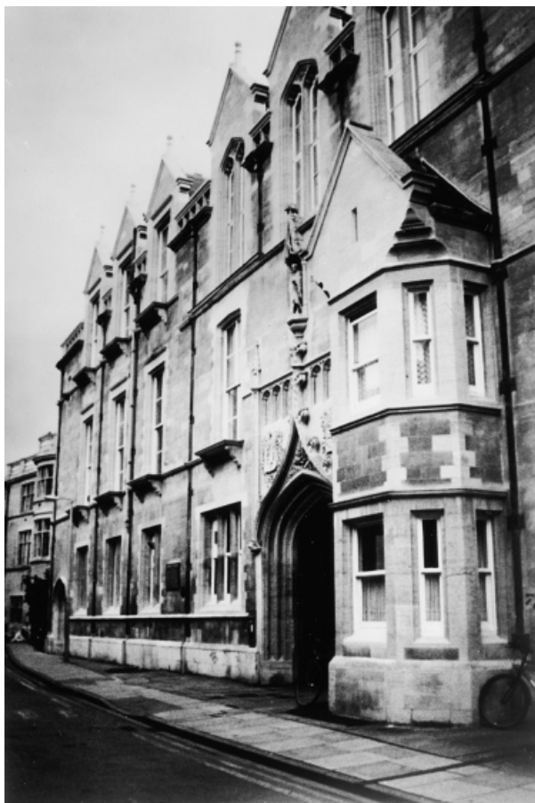
FIGURE 16. The façade of the original Cavendish Laboratory constructed under Maxwell's direction and opened in 1874. It housed some of the most brilliant discoveries in physics made in modern times. It is no longer a physics laboratory, having been replaced in 1974 by a more modern laboratory situated in the suburbs. (Personal photograph.)
