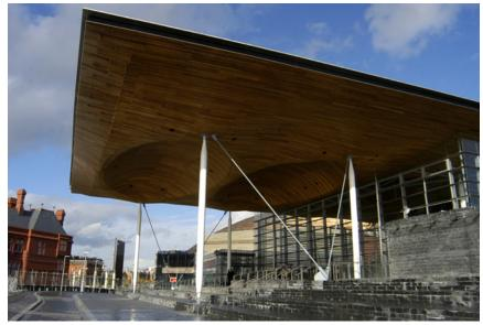
Tie rod base detail. These tie rods use tension to reinforce the cantilevered roof<sup>2</sup>.
