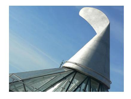
This cowl which sits on the fifth arch back of the roof and raises up 6 meters, making it the largest of its type in Europe. When the wind changes direction, the cowl rotates with the "wind passing the leeward side of the cowl producing a negative pressure" <sup>7</sup> which makes the warm air in the debating chamber below to raise out, naturally ventilating the space. Below the cowl is a lantern (just visible in the image) which allows daylight to enter into the space as well.
