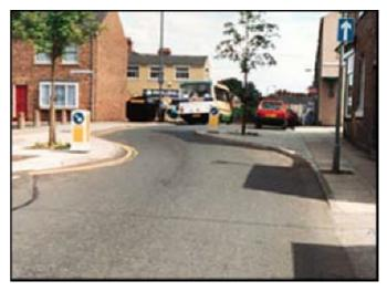
As far as noise is concerned, chicanes will generate less vehicle body rattle than road humps. However, chicanes may encourage more stopping, starting, acceleration and braking noise, and at times these can create a nuisance.
