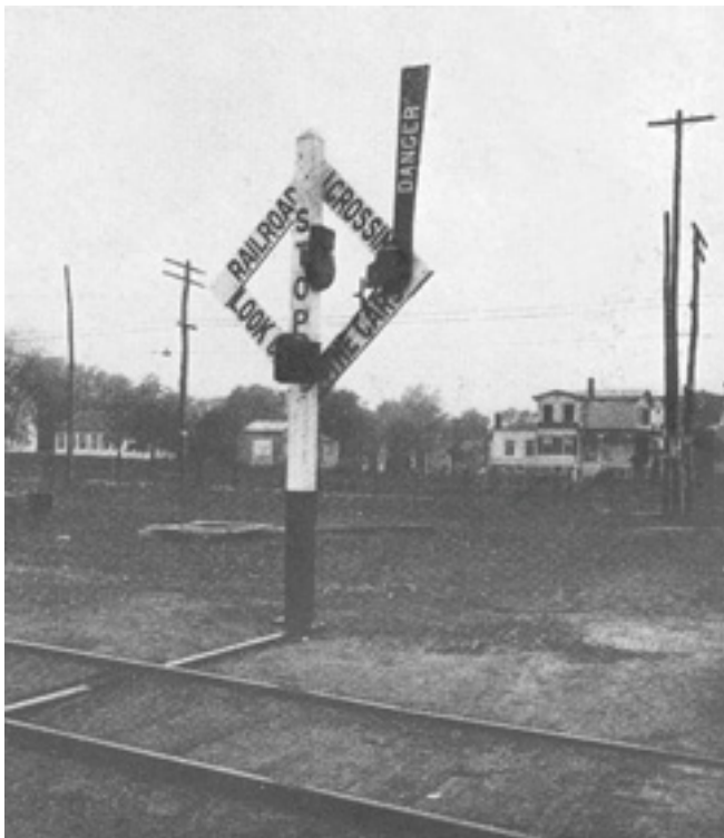
Early Highway Crossing Signal using a Model 2A Semaphore mechanism (1910).
