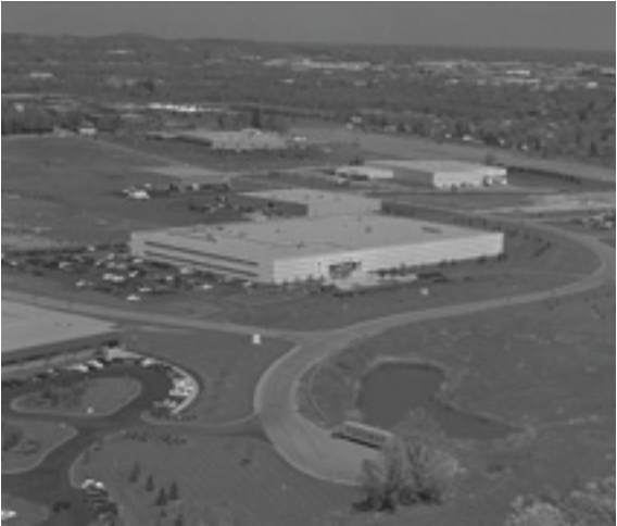
Manufacturing and Office Facility, West Henrietta, NY (1993-Present).
