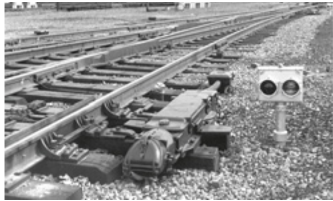
Model 6 Yard Switch Machine (1926).
