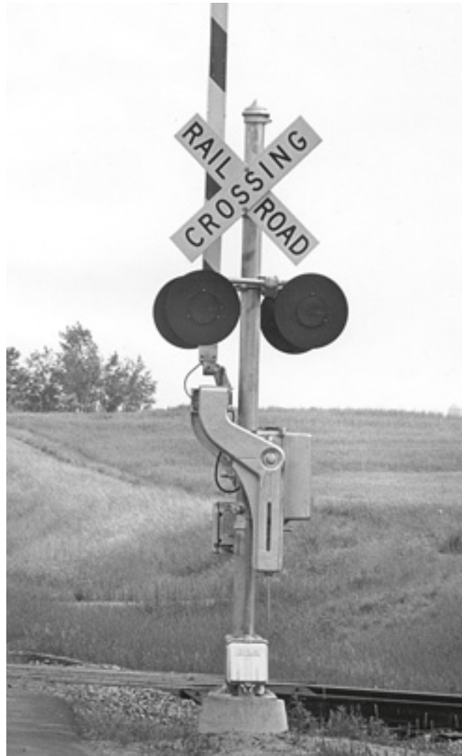
GRS automatic rail-highway crossing with Type D Gate Mechanism.
