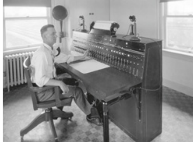
This machine, at Fostoria, Ohio, on the New York Central, controlled the world's first cTc – Stanley to Berwick. The machine is now in the Smithsonian Institute's collection.
