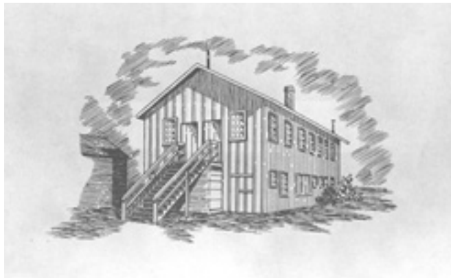
The first dynamic indication electric interlocking machine was made in 1889 by John D. Taylor in this carpenter shop in Chillicothe, Ohio.
