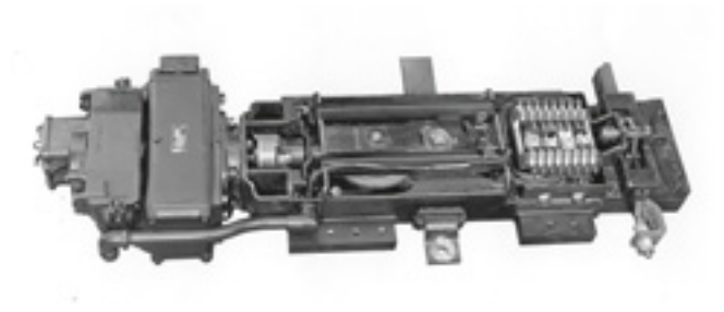
Model 5 Switch Machine (1914).
