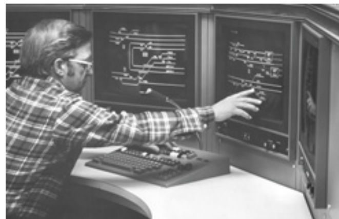
Today's computerized cTc system has a control console with color-video displays of track and traffic conditions and a keyboard to enter commands to the computer.
