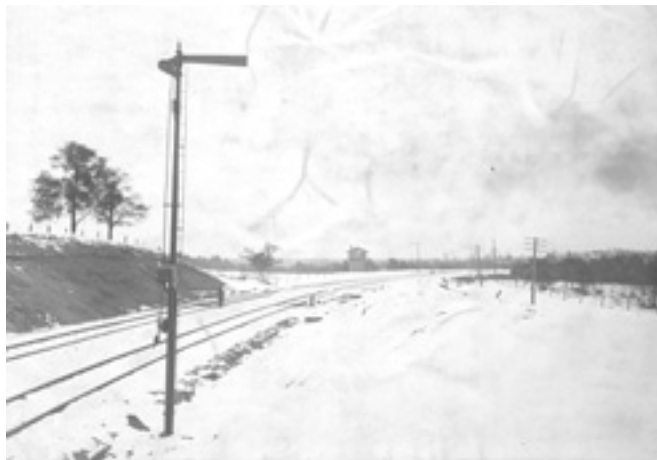
First Taylor Signal Co. electric interlocker was installed at Eau Claire, Wisconsin in 1901 with Model 2 Electric Semaphore signals.
