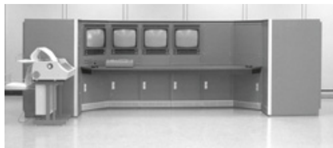
The 534-mile Sishen-Saldahna ore railroad in South Africa is controlled from this color-video display console.
