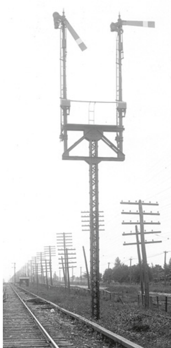
Model 2 Electric Semaphore Signal (ca. 1900).
