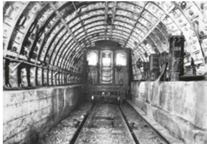
GRS automatic trip stops were installed in 1904 on a New York City subway.
