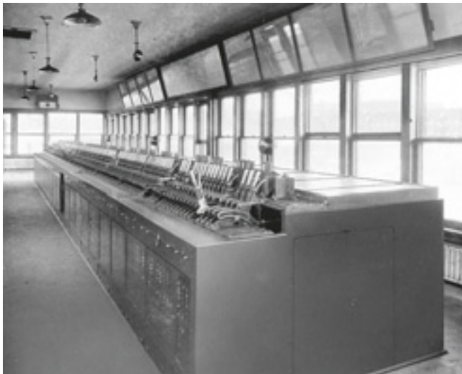
Federal Signal Company electric interlocking machine installed at Utica, New York, on the New York Central Railroad in the early 1920's.
