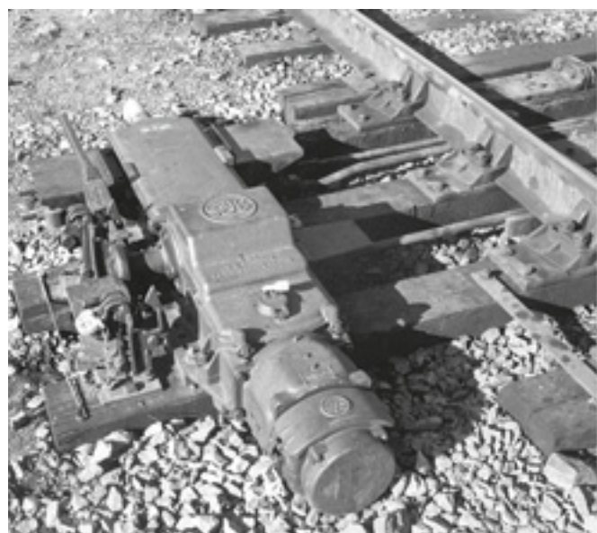
Model 5F Switch Machine (1958).
