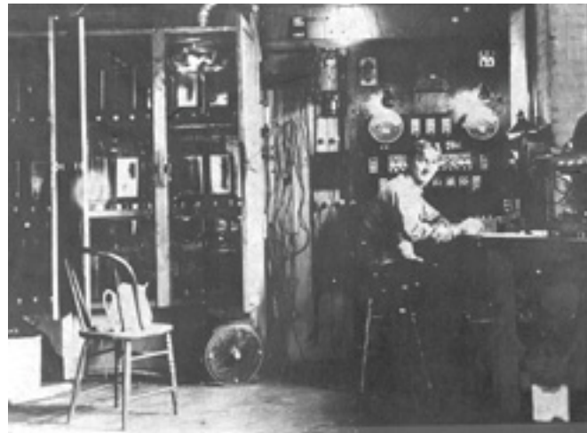
Electrical Laboratory at Taylor Signal Co. in Buffalo, NY (1900).
