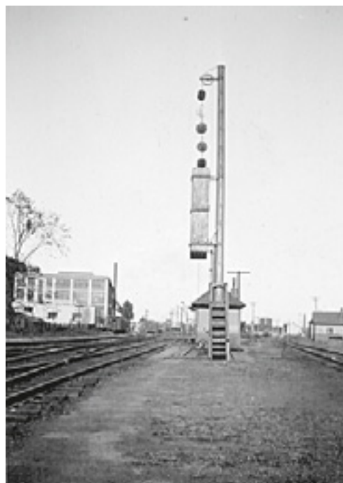
In 1832, ball signals like this one were observed through telescopes from distant block offices.
