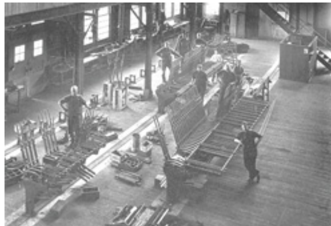
GRS mechanical interlocking assembly department in 1910.
