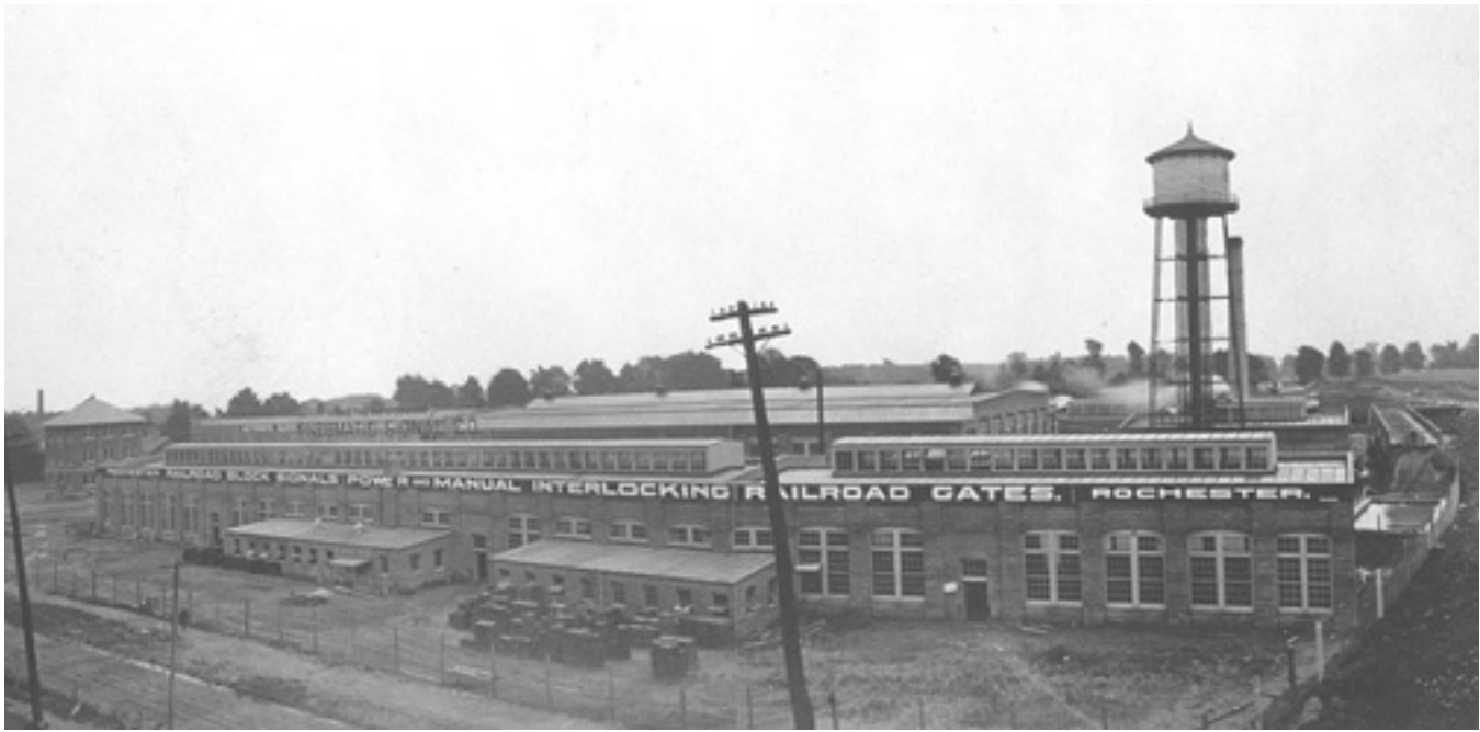
Pneumatic Signal Company plant on West Avenue in Rochester, NY shortly after the formation of the General Railway Signal Company.
