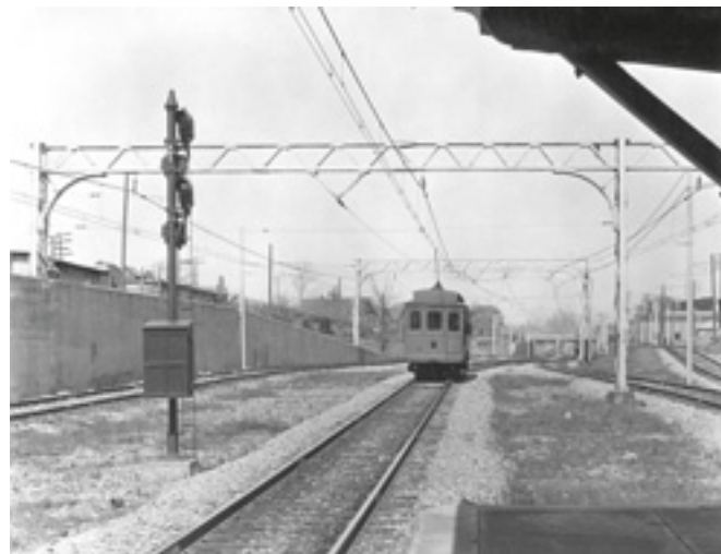
The Rochester, New York subway was equipped with GRS automatic block signal system in 1927.
