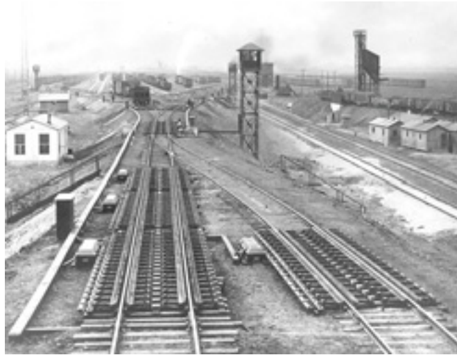
GRS made the world's first installation of electric car retarders of East St. Louis in the Illinois Central in 1926.
