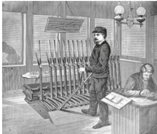
Mechanical interlocking required strong arms and a stout back to operate the signal appliances.
