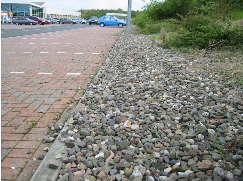
Figure 6.8 – Infiltration SuDS (Permeable Paving and Filter Strip)
