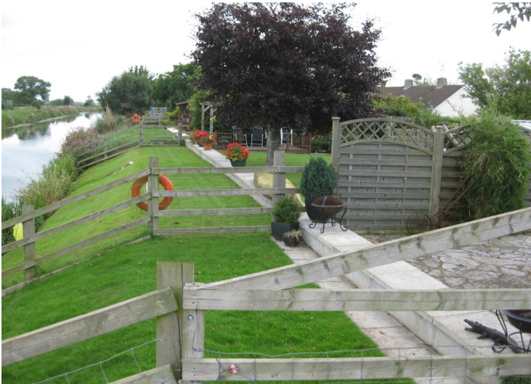
Figure 6.1 – Raised Earth Embankment
