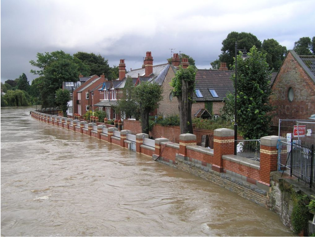
Figure 6.2 – Raised Flood Wall
