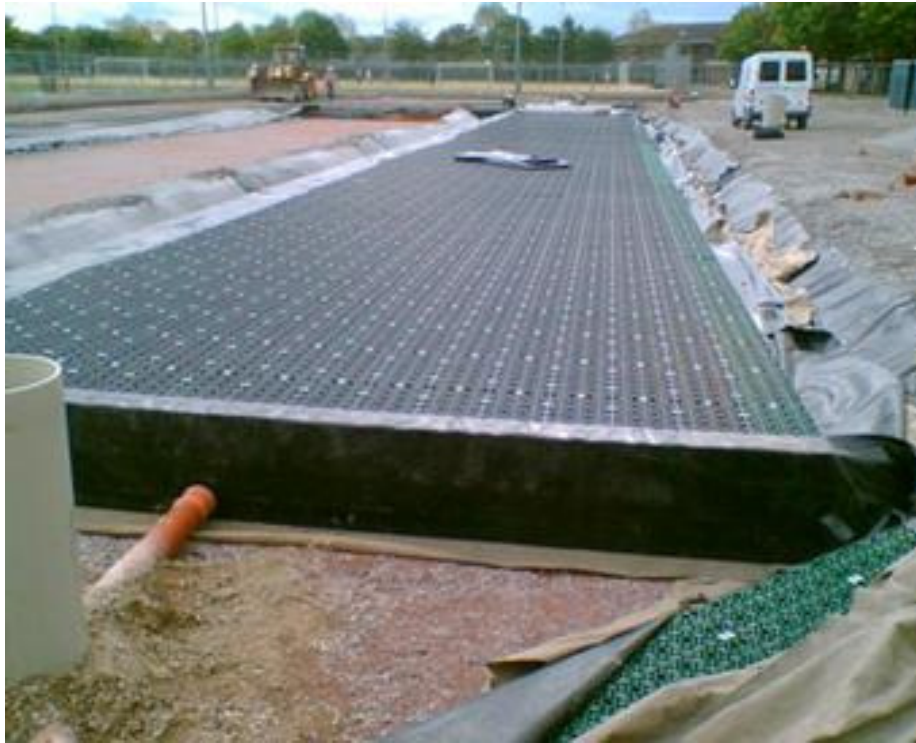
Figure 6.13 – Permeable Paving installation
