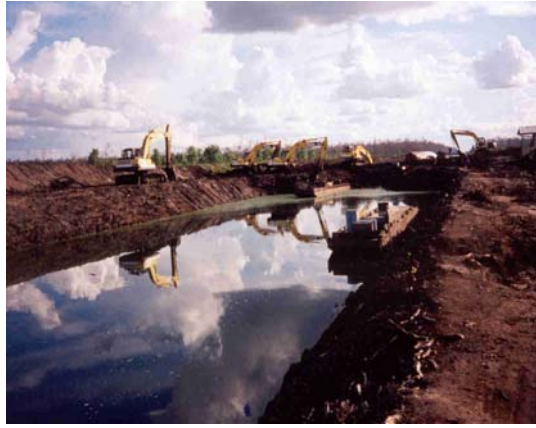
(b) Channel construction in 1997, Block C.
