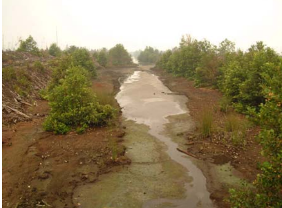
Figure A 2-7: subsiding secondary channel
