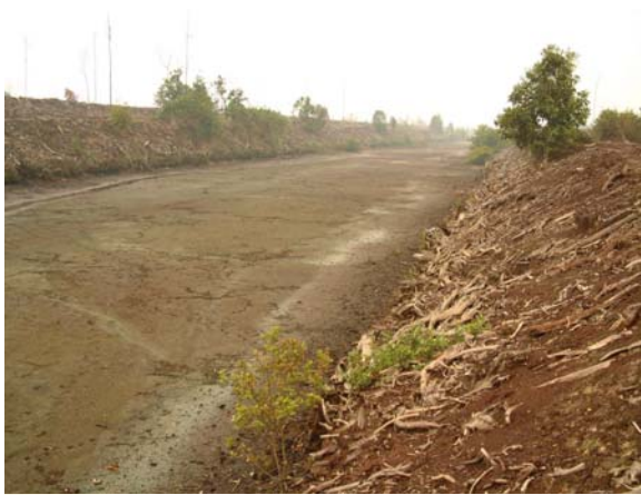
Figure A 2-6: dried out, inoperable primary channel
