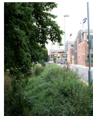
Sustainable Urban Drainage System at BedZed
