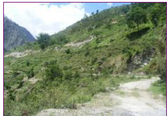
Approach Road to Langsi Adit (Old road route to Badrinath below NH 58)
