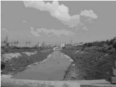
Fig.3 Open Drain – Mattikere Tank
