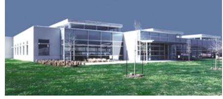
Exposed concrete floors are located in the lobby, kitchen and corridors. Glazed aluminum curtain walls and clerestory windows provide natural light. Kirksey Architecture was able to make minor adaptations to conventional design methods to accomplish the finished project – the result of which was a straightforward, cost-effective and energy-efficient design.
