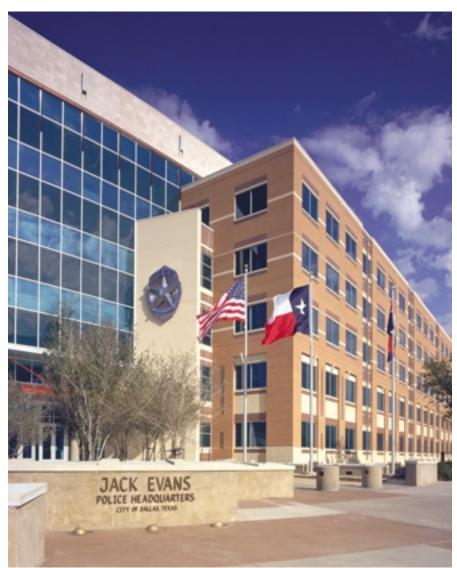
brick veneer, cast stone on metal studs, curtain wall, ribbon windows and punched windows all with low-E glazing. The building also includes an exterior courtyard on level two and a skybridge connecting the new facility to an existing parking garage.
