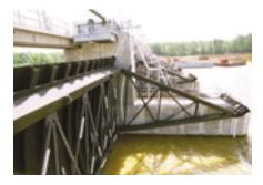
Installing the elaborate series of gates was a challenge. The two pie-shaped sector 63- ton gates are each 30 ft. by 30 ft. and made of A36 steel. The gates were jacked into place.
