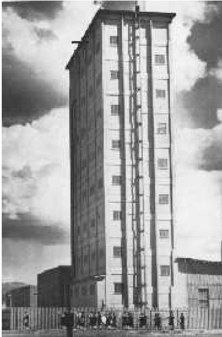
Figure 5: The Trail Heavy Water tower in the late 1940s (B.C. Archives and Records Service Cat. No. NW669 C733 V.30-32/1)
