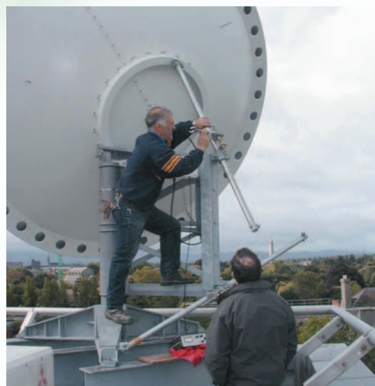
Installation of the 4-metre antenna
