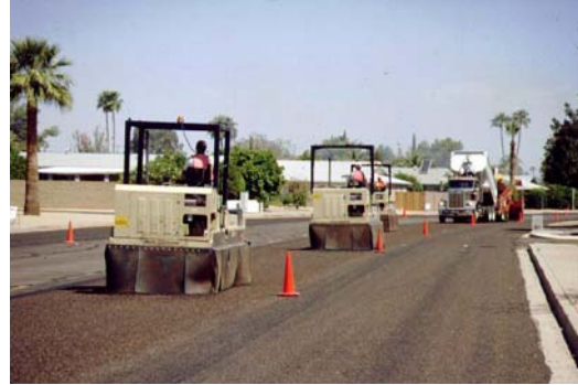
Figure 4-4: Rubber-Tired Rollers With Skirts On Chip Seal
