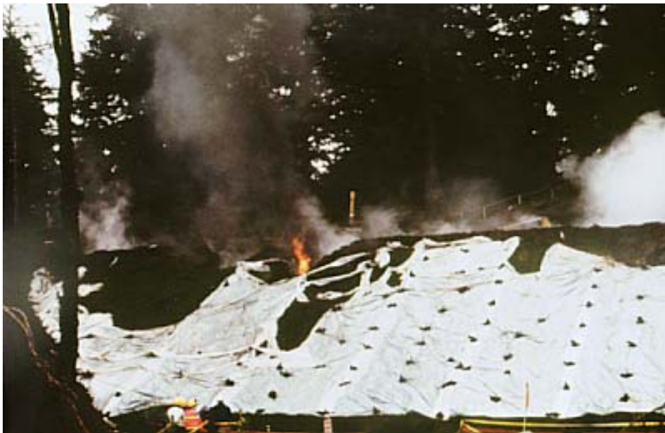
Figure 2. SR100 Ilwaco Fire During Embankment Removal
