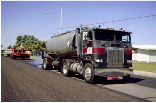
Figure 2-5: Chip Seal Train
