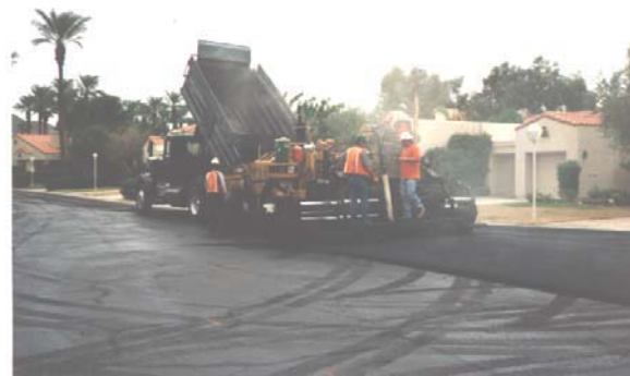
Figure 4-1: Unloading RAC-G Into Paver Hopper
