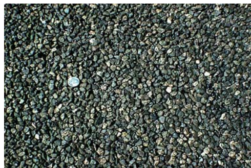
Figure 4-6: Finished Chip Seal Before Applying Fog Seal and Sand
