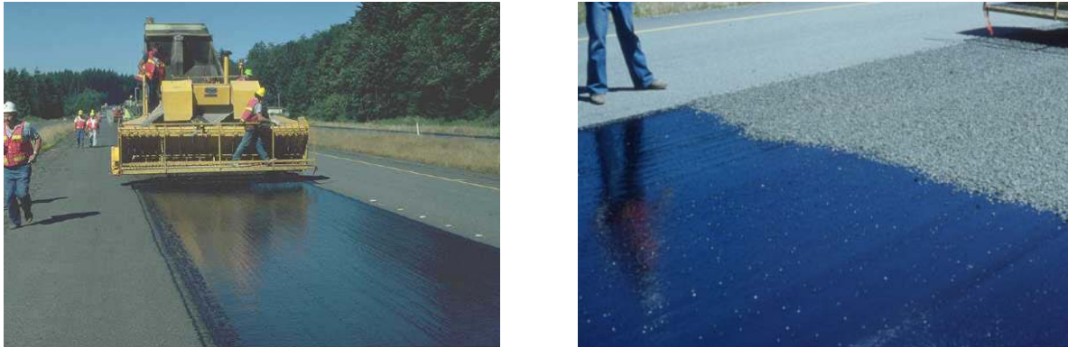
Figure 15. Chip Seal Construction
