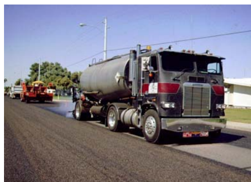
Figure 4-2: Chip Seal Train
