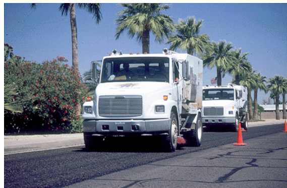
Figure 4-5: Sweeping Chip Seal To Remove Loose Cover Aggregate
