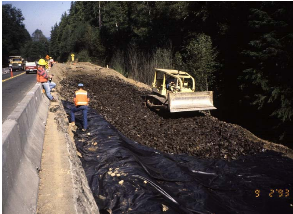
Figure 1. Lightweight Tire Fill Construction
