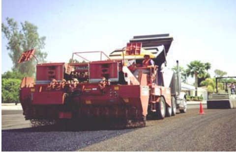
Figure 4-3: Spreading Precoated Aggregates
