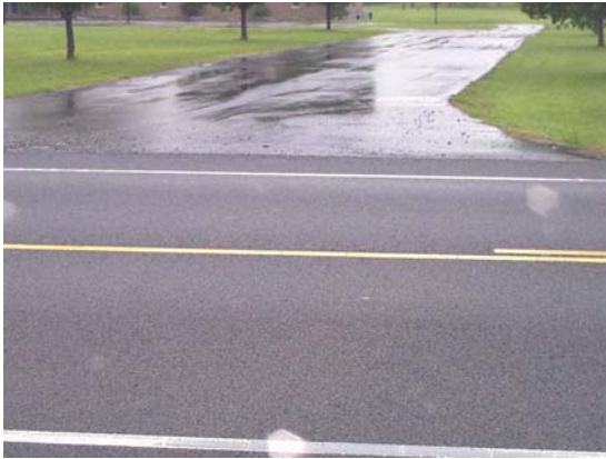
Figure 2-4: Free-Draining RAC-O Next To DGAC
