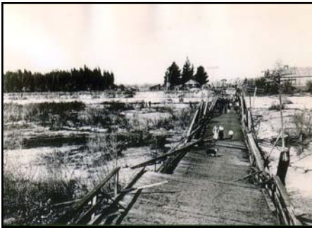
Flood damage- Rio Honda River c1914
