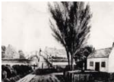
Five Bells Lane Bridge
