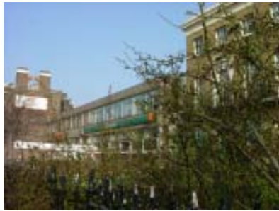
Poor quality Post Office building
