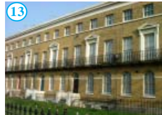
Hatcham Terrace, 207-229 Grade II listed, c1840
