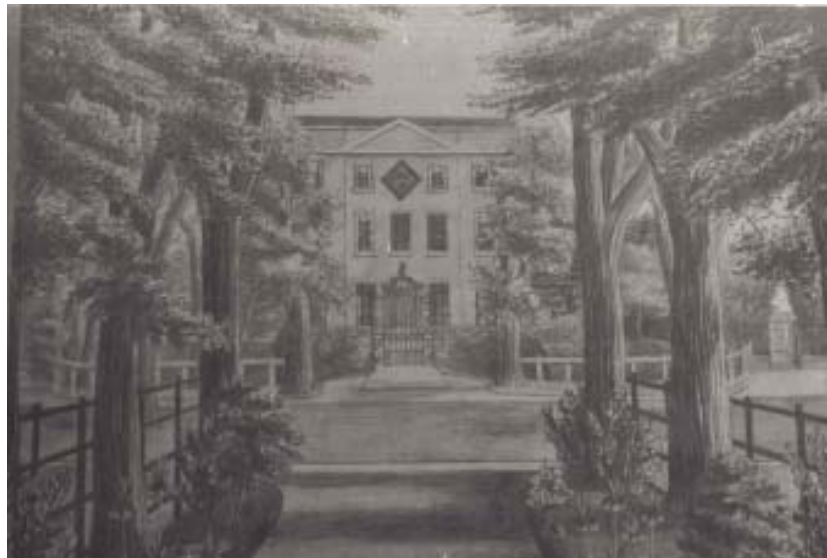
Hatcham House which was demolished in 1869
