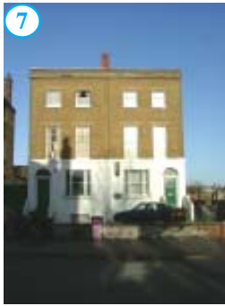
371-373 Queens Road, Grade II listed, c1840
