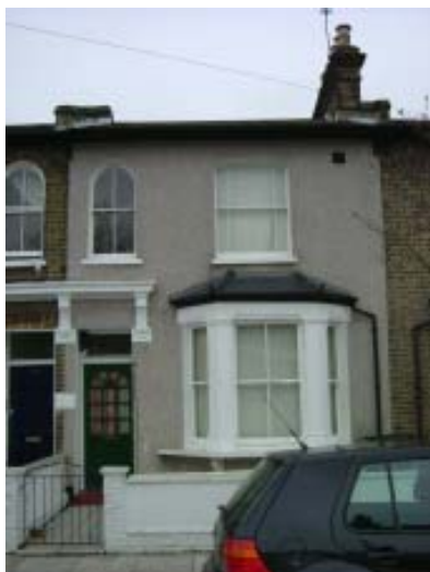
Covering brickwork with pebbledash or other coatings obscures brickwork which is otherwise attractive in itself. Such interventions also severely disrupt the unity of the terrace
