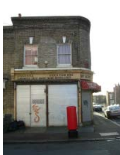
Shop at the corner of Egmont Street and Camplin Street
