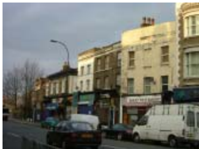
Poor quality shopfronts, signage and poor maintenance of the upper storeys
