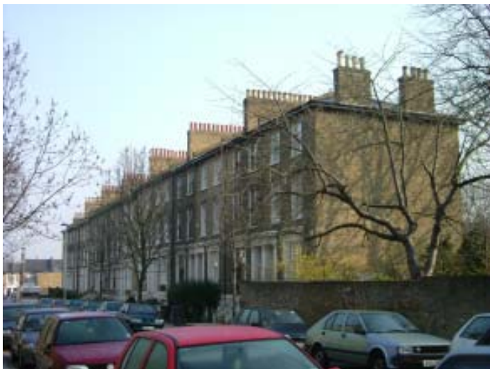
View along Nettleton Road
