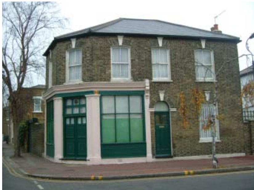
Converted shop in Barlborough Street
