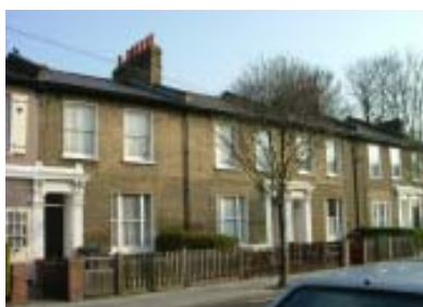
View along Hatcham Park Road
