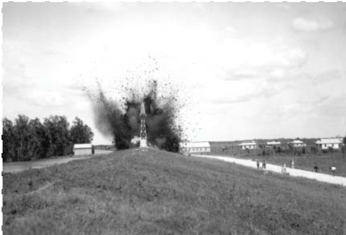
With MRC approval, Gov. Simpson gave the "go ahead" to dynamite the Caernarvon levee below New Orleans to create an artificial crevasse during the 1927 flood. The effort not only saved the city, it also blew away the "levees only" policy of the MRC.
