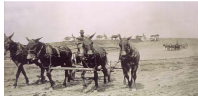
Early levee construction
