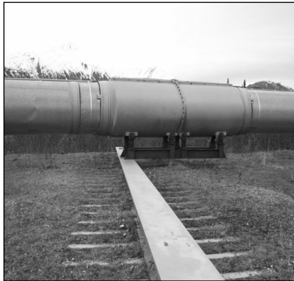
Figure 6. Post-earthquake shoe location on grade beam prior to re-centering.
