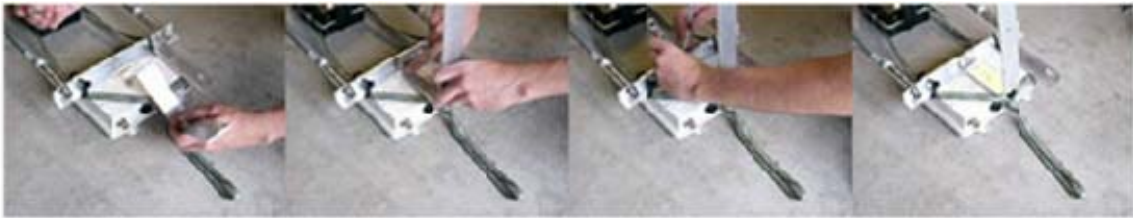
Figure 21. Installing the camera bracket
