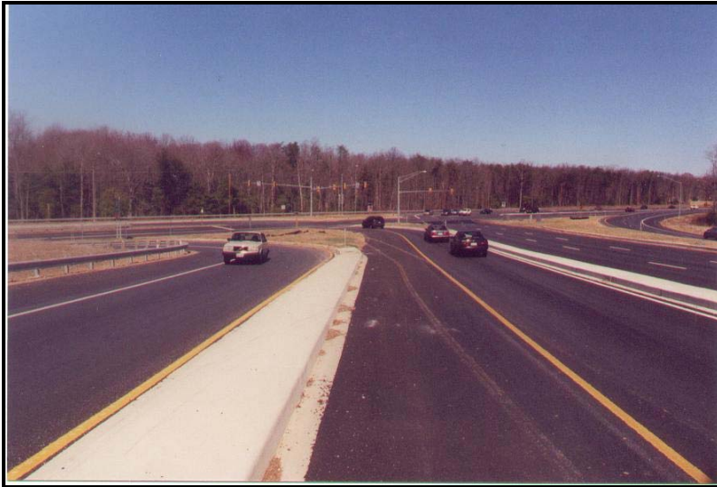
Figure A.4.7. MD 228 Westbound -- View of Intersection
