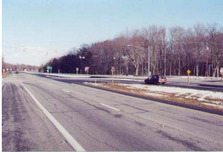
Figure A.2.1. Superstreet Intersection in Kent County, MD (Photos by Cipriana D. Thompson)
