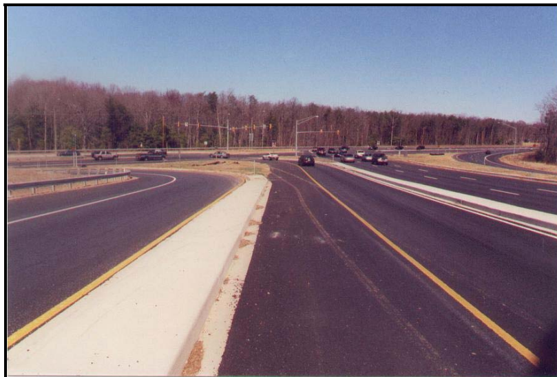
Figure A.4.6. MD 228 Westbound -- View of Intersection
