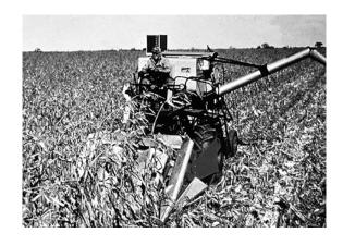
"When Gleaner got started in self-propelled combines, they sold the machines on their center-line design, the down-front threshing cylinder, the two-fan cleaning system and the simplicity," says Ross Yohn, a retired Gleaner engineer who started with the company in 1957. "Those were features that carried all the way through Gleaner's history."
